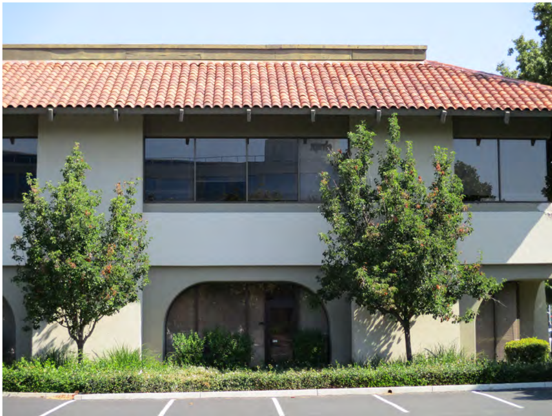
Photo 2: Close up view of the architectural style of the existing office buildings.
