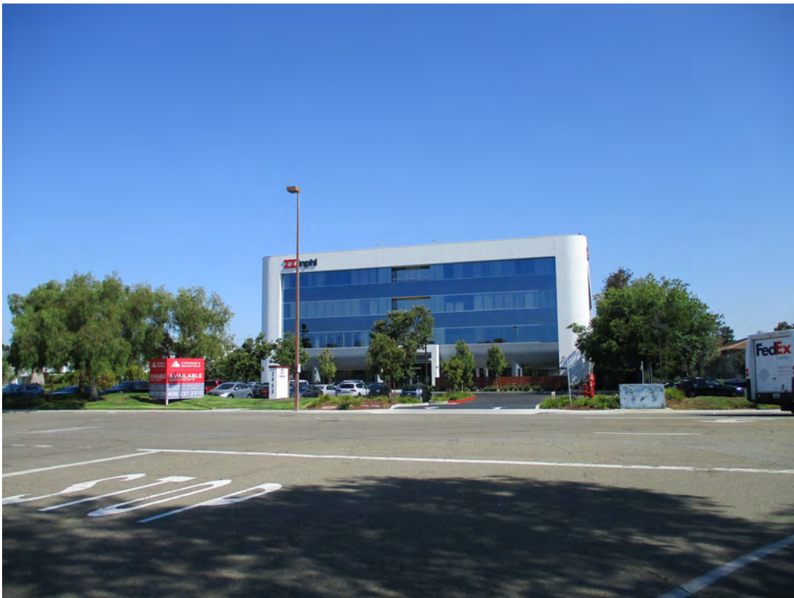
Photo 4: View of the four-story office building across Bunker Hill Lane, north of the project site.
