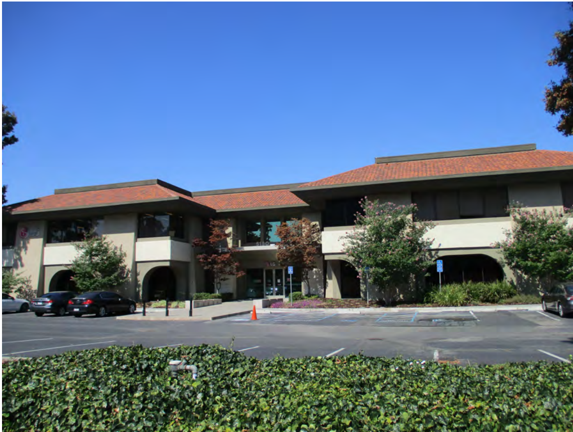
Photo 1: View of the existing offices on the project site.
