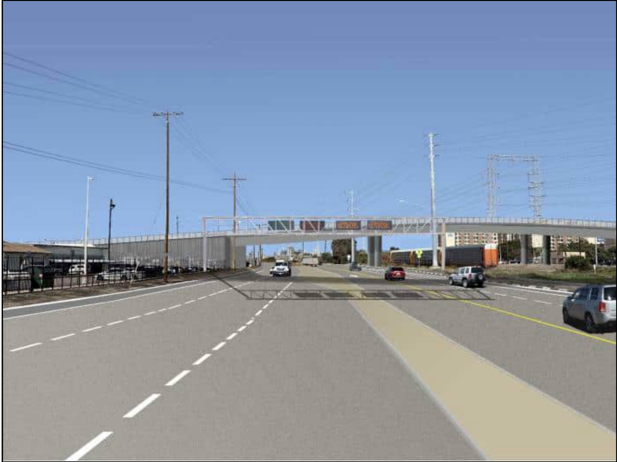
Figure 2-10: Key View 2 Proposed Condition – Build Alternative (Vesta Street Bridge Option 2, Precast Wide-Flange Girder Structure with Columns)
