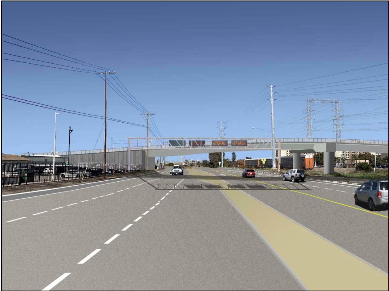
Figure 2-9: Key View 2 Proposed Condition – Build Alternative (Vesta Street Bridge Option 1, Cast in Place Box Girder with Outrigger Bent)
