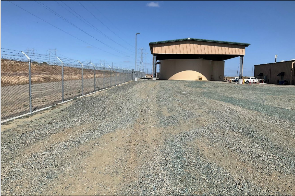
Figure 4-3 Overview of Project area from southeast end of proposed trench, facing northwest.
