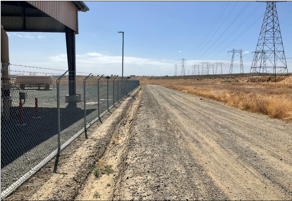
Figure 4-2 Overview of 50-foot buffer, outside of Project area. Southwest end of the Project area, facing southeast.
