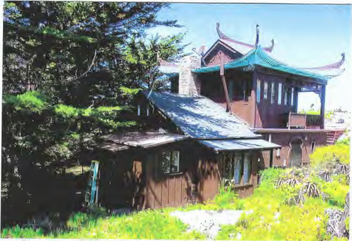
Photo #3. Looking SW at the rear (NE) elevations, note, inappropriate one-story 1950s addition at left, Kent Seavey, Dec., 2021.
