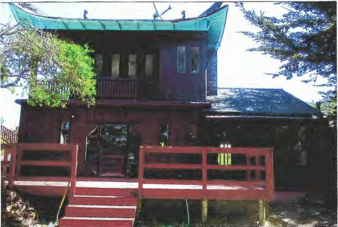
Photo #2. Looking North at the SW side-elevation, note existing raised deck, & addition to right, Kent Seavey, Dec., 2021.
