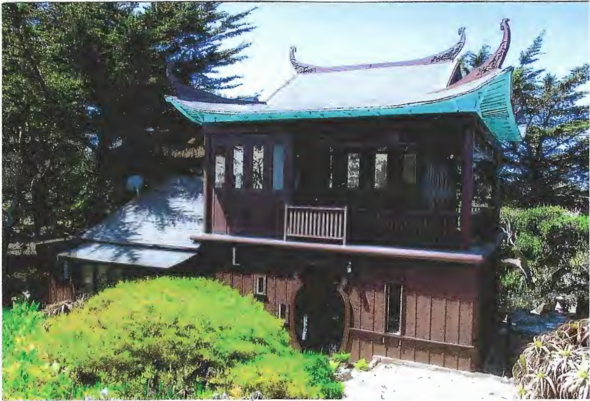
Photo #1. Looking SE at the NW side-elevation, note one-story 1950s addition at left. Kent Seavey, December, 2021.
