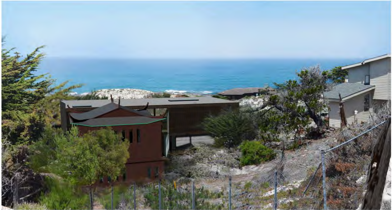
View from the east looking west
