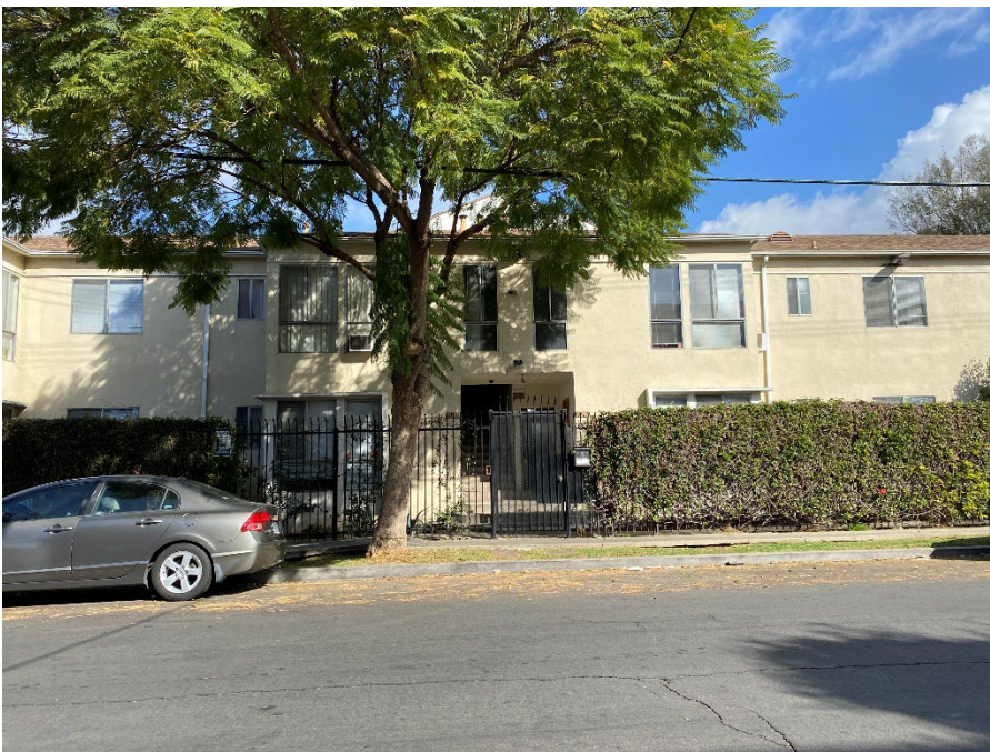
South façade of south residential building looking north from Lexington Avenue.
