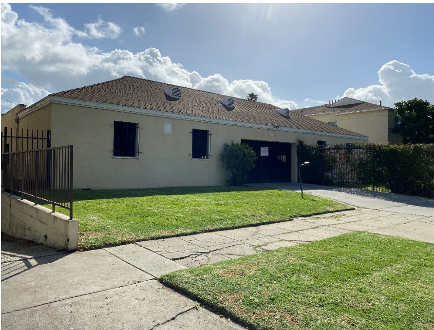
West garage entrance looking southeast from Lodi Place.
