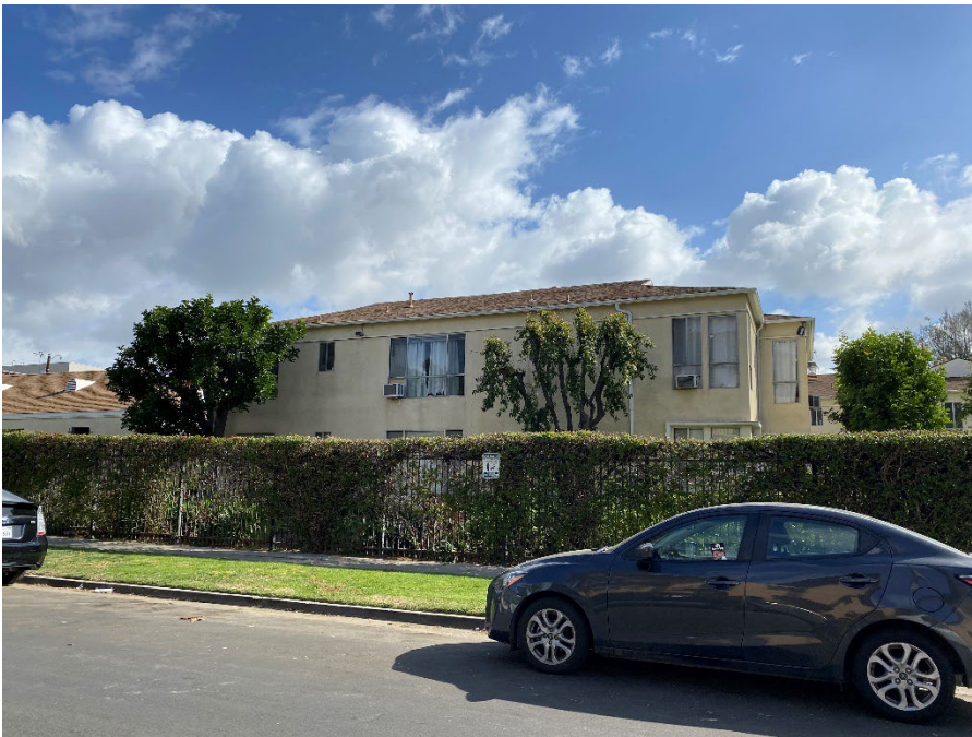
West courtyard building looking east from Lodi Place.
