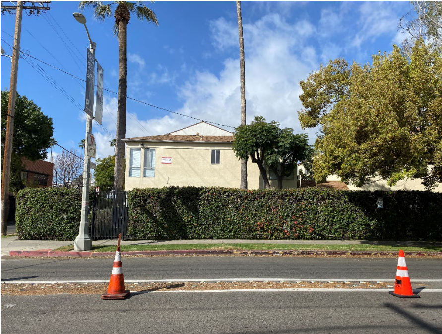
East façade of south residential building looking east from Gower Street.
