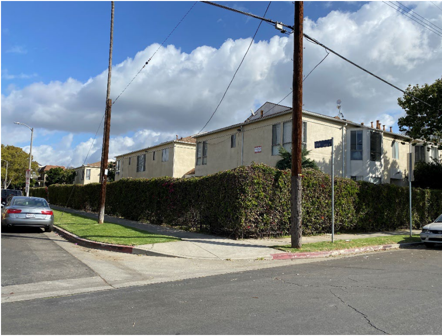
South residential building and west courtyard building looking northeast from Lexington Avenue and Lodi Place.
