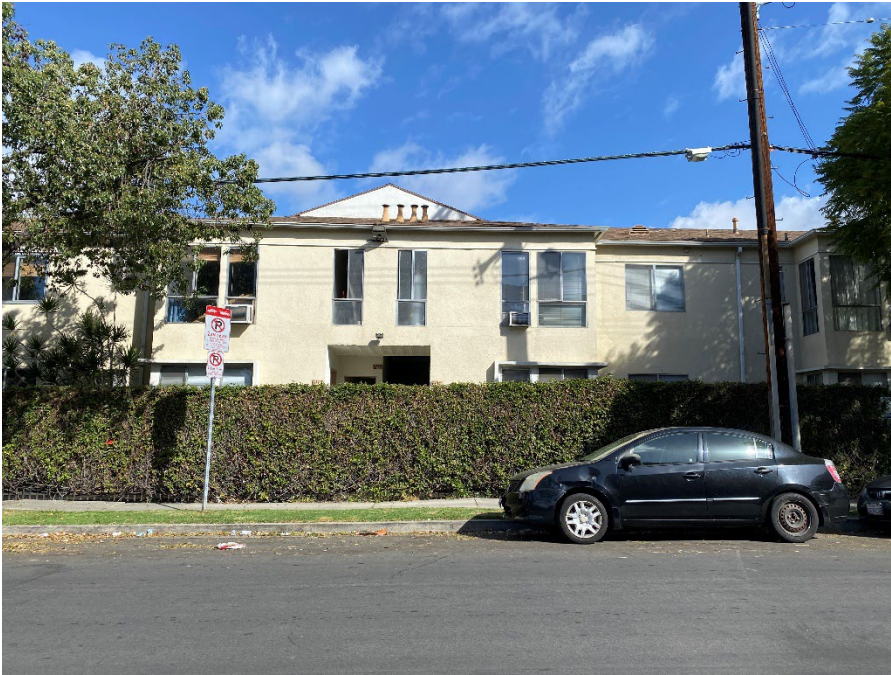
South façade of south residential building looking north from Lexington Avenue.
