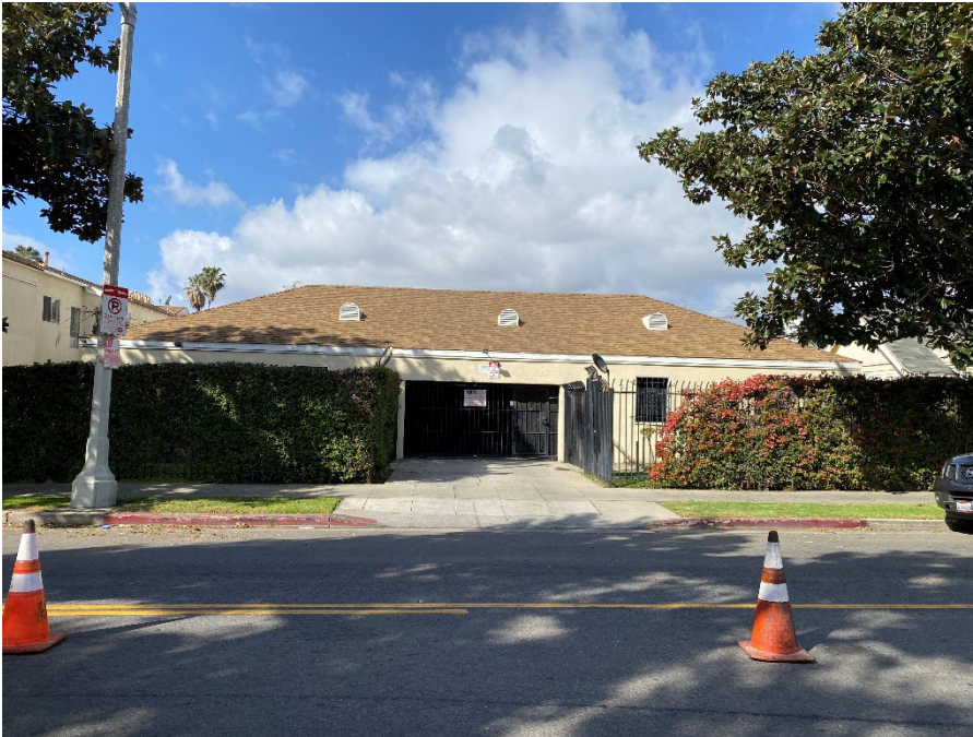
East garage entrance looking west from Gower Street.
