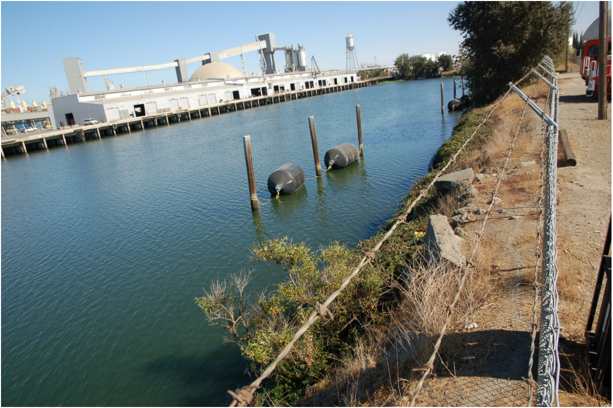
Photograph 3 View from the Project Site, Looking Southeast
