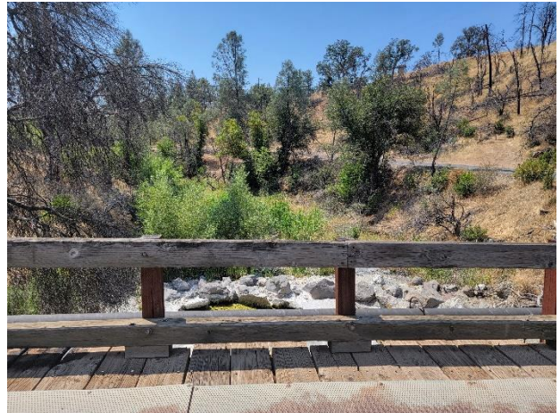
Photo 4: Standing on the center of the Wolf Creek Bridge looking downstream.
