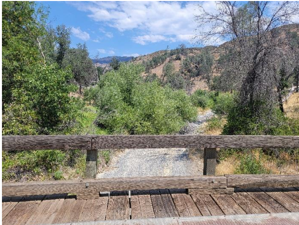
Photo 3: Standing on the center of the Wolf Creek Bridge looking upstream.
