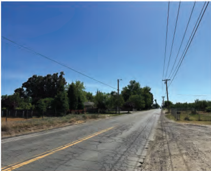
View east along Service Road near Central
