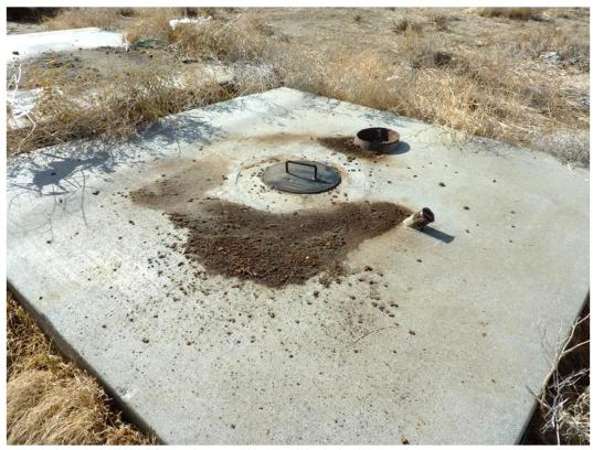
E-11. Concrete pads for water well in SEC of site. Steel plate over well welded in place; status of well casing (sealed or open) unknown (12/15/2021).
