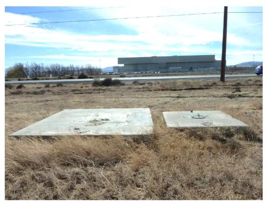
E-14. Looking south at concrete pads for water well inside southern site boundary with AFP 42 (Plant Site 4) in background. Steel plate over well welded in place; status of well casing (sealed or open) unknown (12/15/2021).
