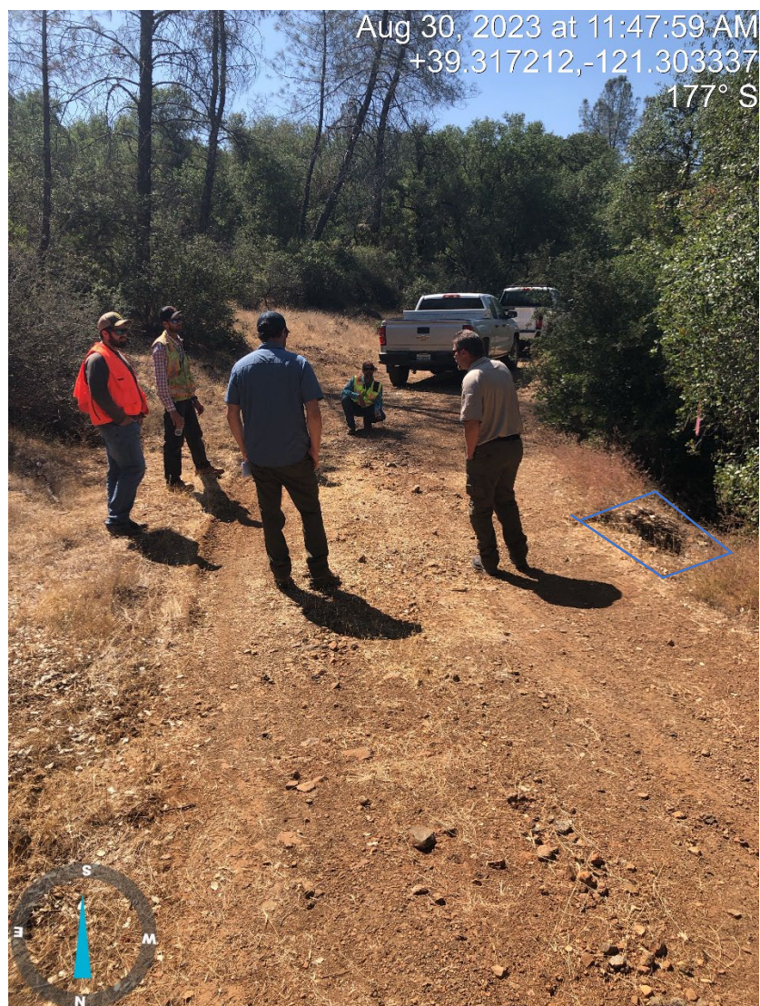
Location 5: Low point in road that stays wet after rain events. For Phase 1, rock will be hand stacked to an eroded area on the edge of the road (area in blue polygon). Phase 2 work will include a plan for a more long-term stable solution.
