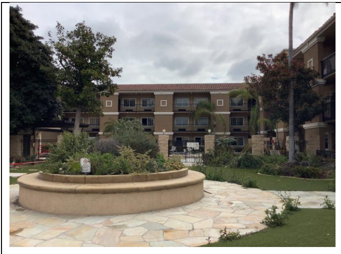
Photo 4. Courtyard, facing east
