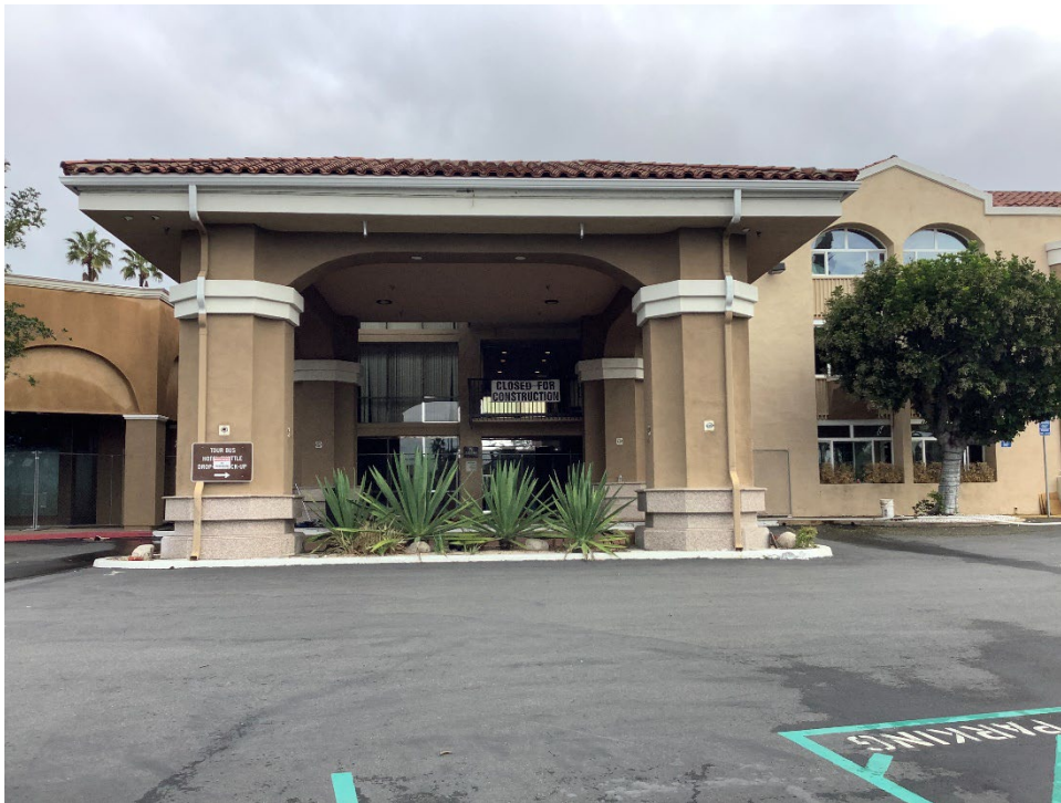
Figure 5-2. Entrance carport, facing north.
