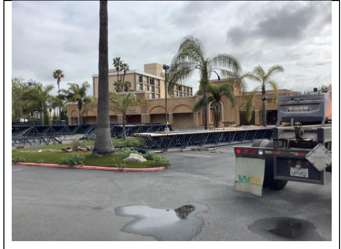
Photo 3. West elevations of commercial section with the tower block behind, facing northeast
