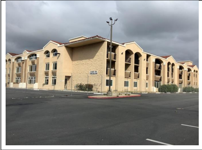
Photo 2. South and east elevations of the original hotel, facing northwest
