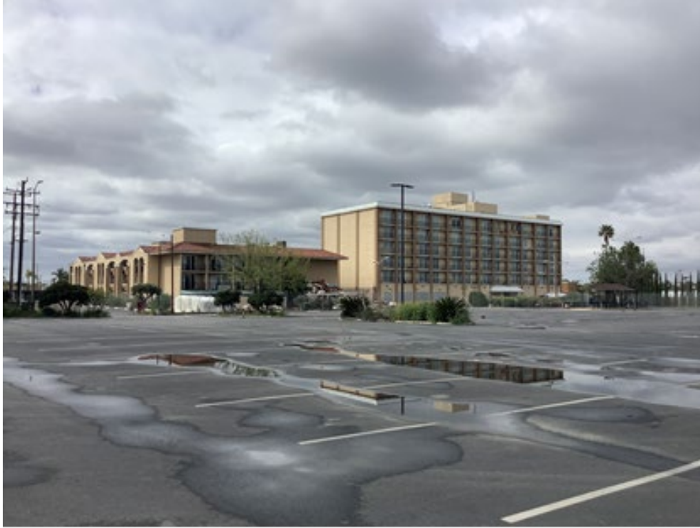
Figure 5-1. Overview of the Hotel Fullerton, facing northwest.
