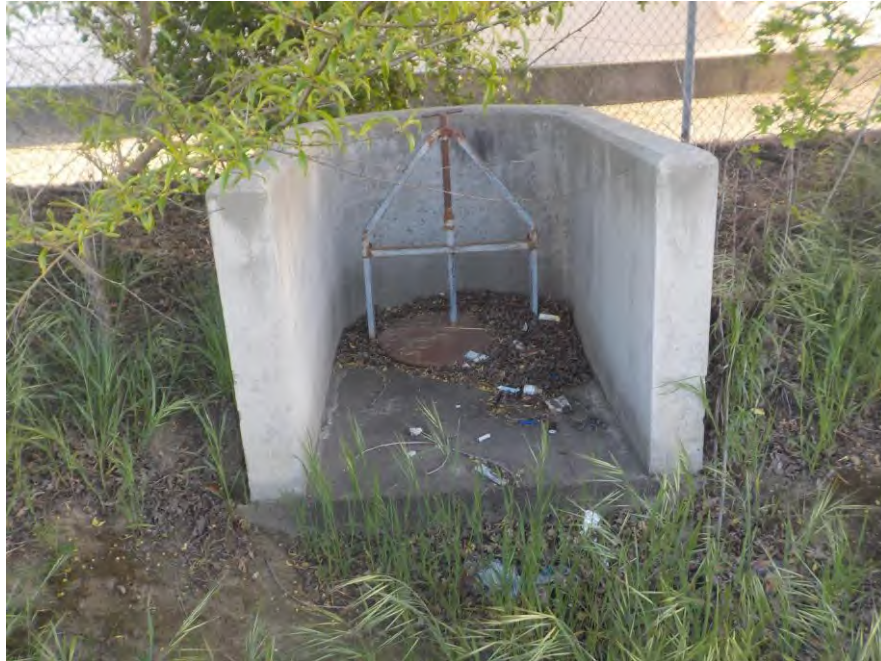
Photograph 23 – Additional Drainage/Irrigation Feature #2 From North, Facing South
