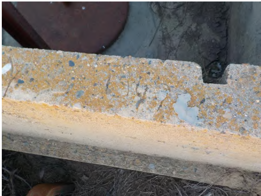
Photograph 22 – Additional Drainage/Irrigation Feature #1 from North, Facing South
