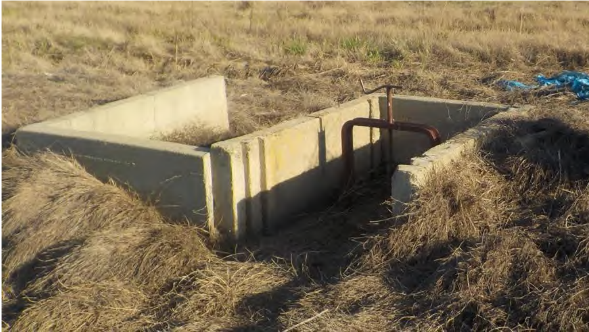
View of Drainage/Irrigation Feature 3, from Northwest, facing Southeast, Taken 4/14/23, Photo # 616
