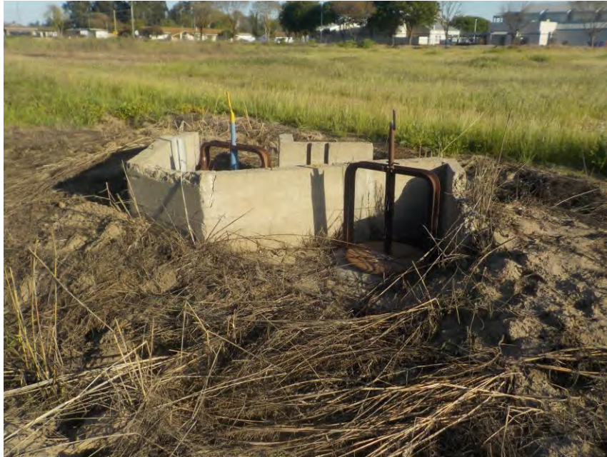
Photograph 13 – Drainage/Irrigation Feature 2, within La Coste Lane Parcel 1 North Mar Basin, from Northwest, Facing Southeast
