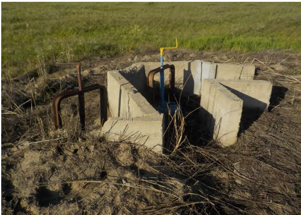
View of Drainage/Irrigation Feature 2, from Southwest, facing Northeast, Taken 4/14/23, Photo # 597
