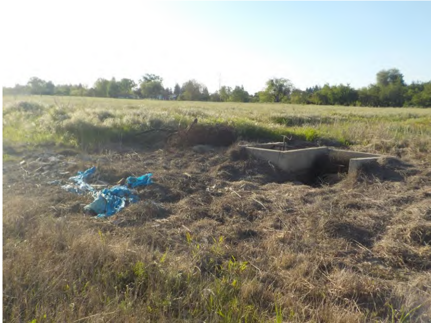
Photograph 17 – Drainage/Irrigation Feature 3, within La Coste Lane Parcel 1 North Mar Basin, showing Rubble Pile to South, from Southeast, Facing Northwest
