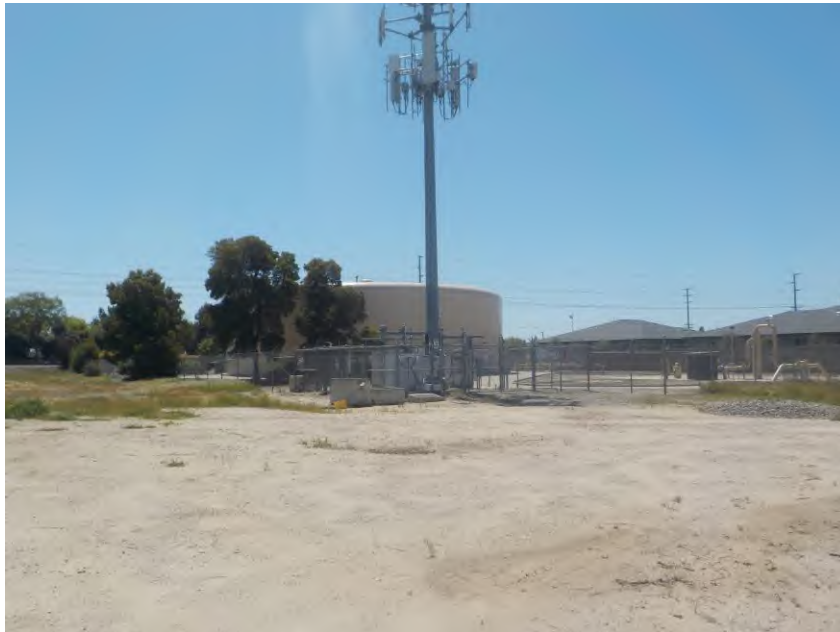
Photograph 4 – View of Well 65 Mar Basin Laydown Area, taken from Northwest corner, facing Southwest
