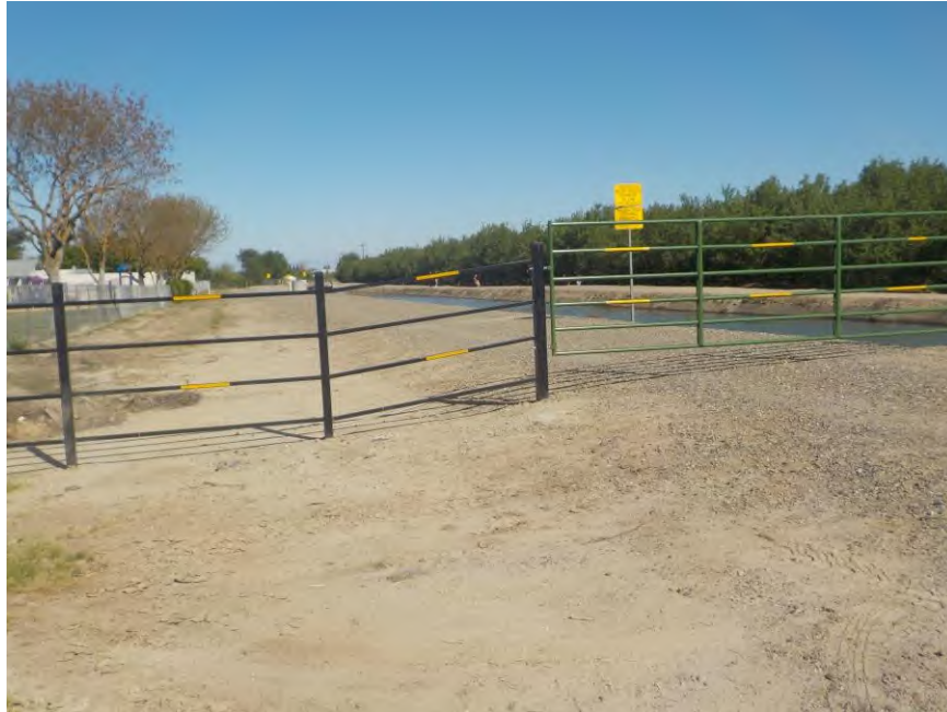
Photograph 25 – View of Proposed Pumphouse Area for La Coste Field 1 and 2 Basin Areas
