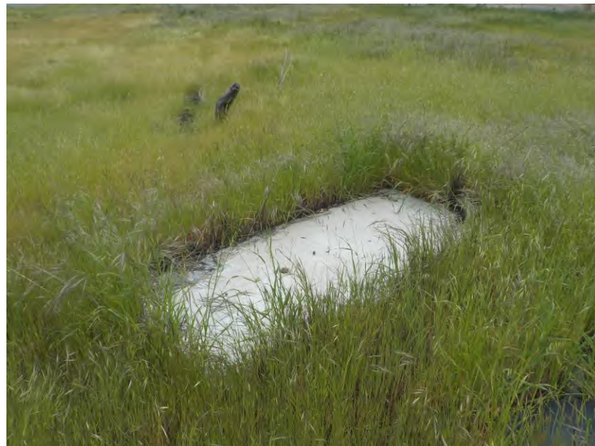
Photograph 8 – View of Concrete Slab within Proposed Pumphouse Area for Ustach Park Mar Basin, facing Southeast
