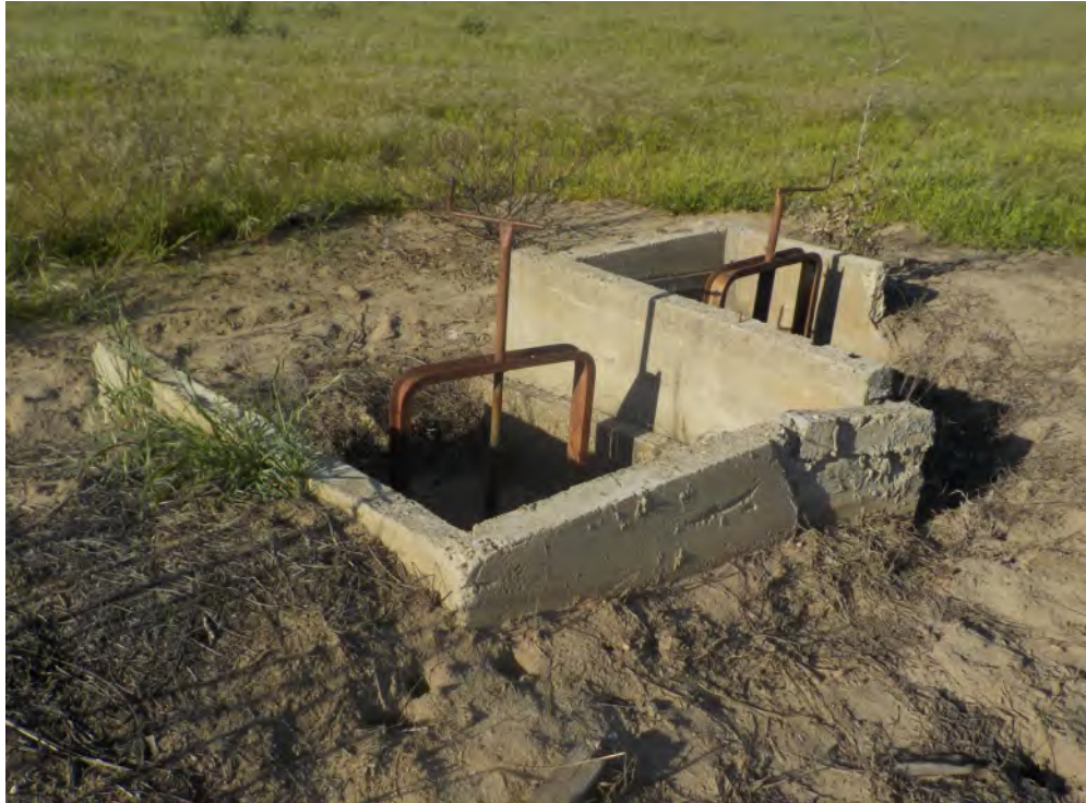
View of Drainage/Irrigation Feature 1, from Southwest, facing Northeast, Taken 4/14/23, Photo # 583
