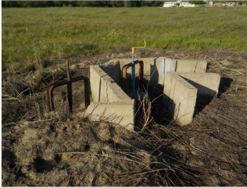
Photograph 11 – Drainage/Irrigation Feature 1, within La Coste Lane Parcel 1 North Mar Basin, from Northwest, facing Southeast
