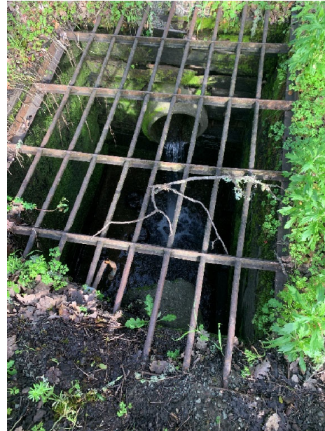
Photo 4. Buried drainpipe from OW 1 enters the storm drain (March 7, 2024).
