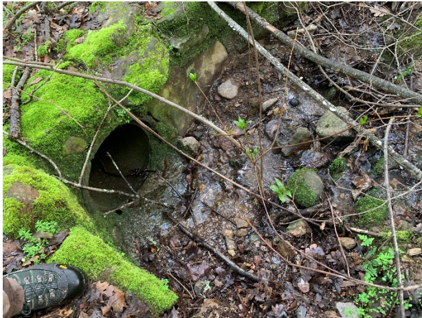
Photo 3. OW 1 enters a buried drainpipe (March 7, 2024).
