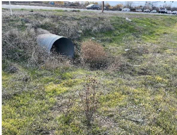
Photograph 6. Existing culverts on the site
