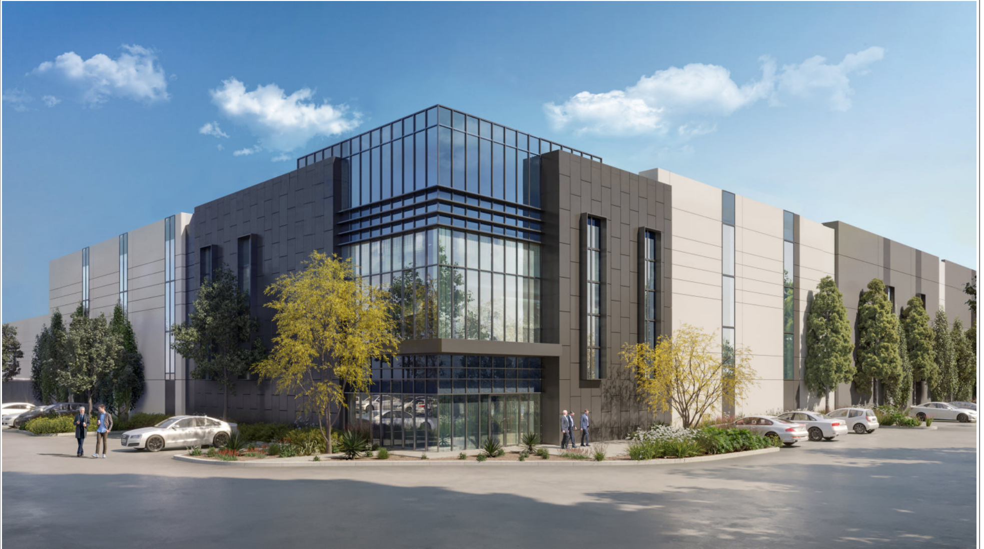
Looking Northwest Towards the Southeast Corner of Building
