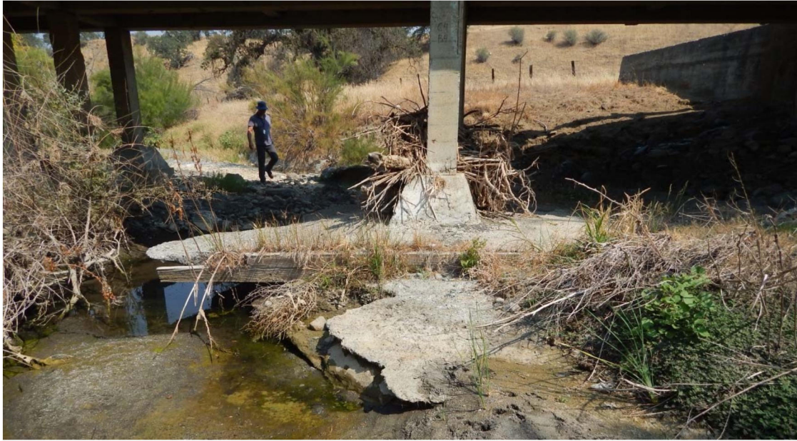
Figure 18: Looking upstream through the bridge showing significant debris caught on the pier and undermined concrete paving
