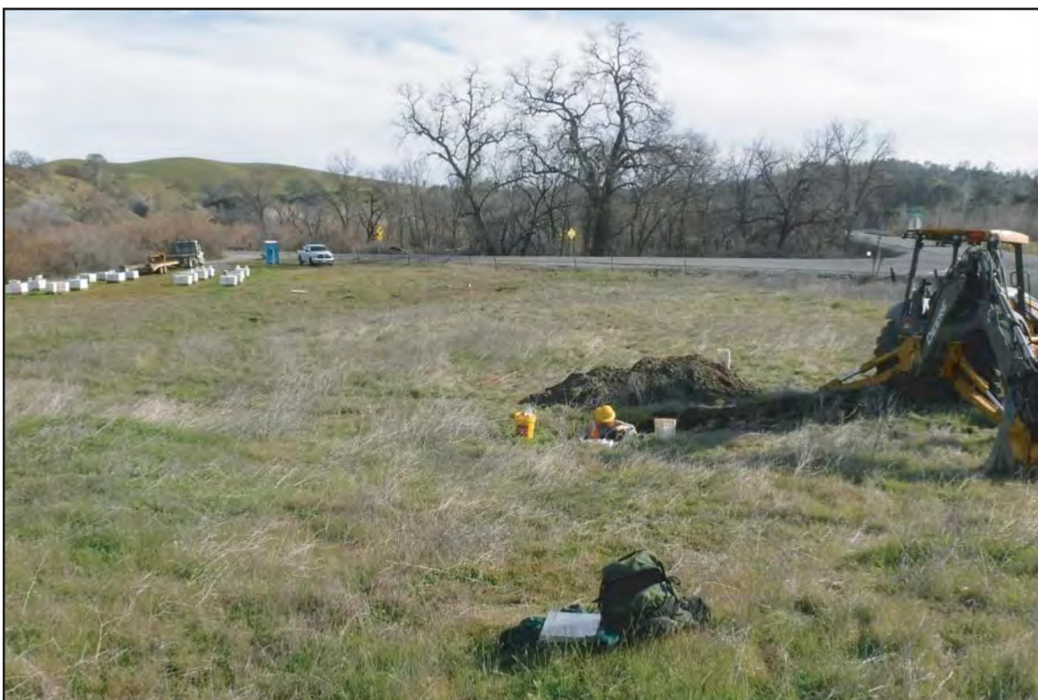
Figure 3. Overview Photographs of Trenching Operations at Trench 2 (Above) and Trench 4 (Below).
