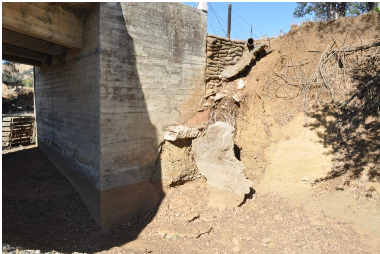
Figure 11. Undermining and scour at Abutment 2 of the existing bridge.
