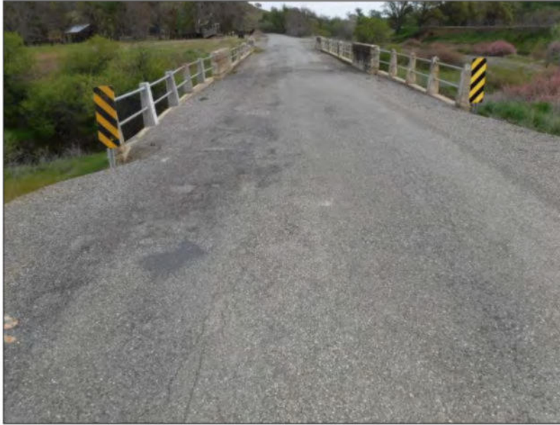
Figure 1. Overview of APE, with the Branch Salt Creek Bridge in foreground, view east.
