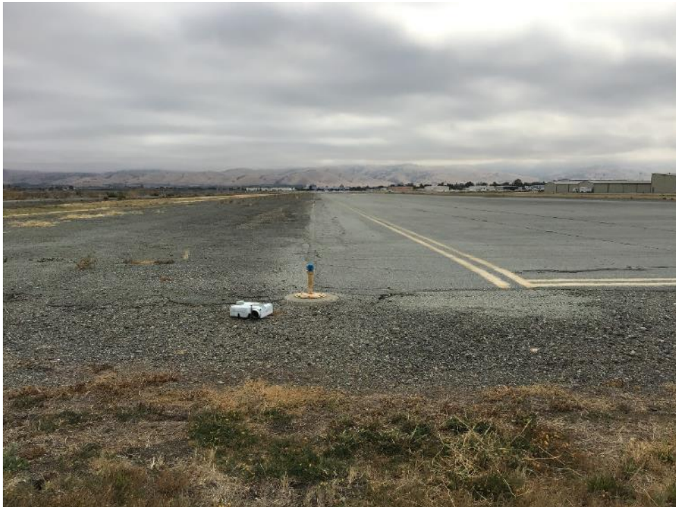
Photo 4. Runway 6 hardscape to be removed. Taken facing east.
