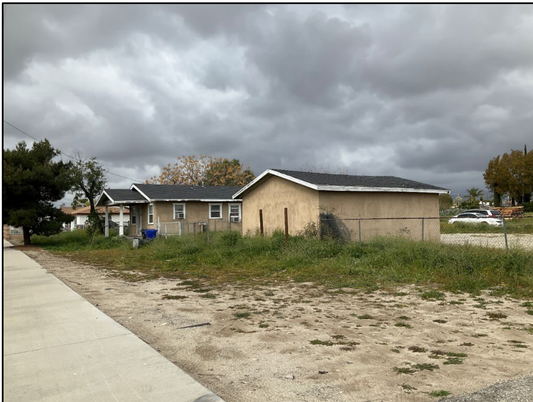
Photograph 4. Historic residence and garage on 17764 Merrill Avenue, facing northwest
