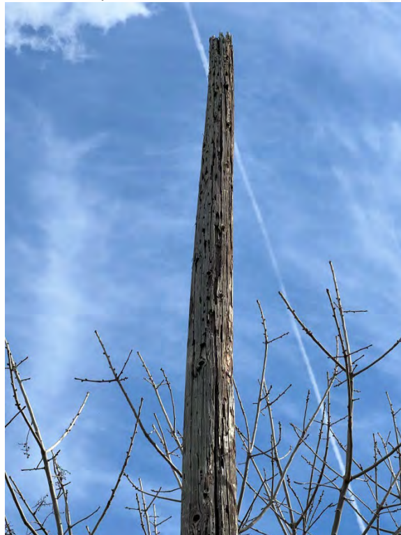
Photo 12. Top of an unmarked electricity pole with woodpecker damage located on the northeast quarter of APN 441-382-04
