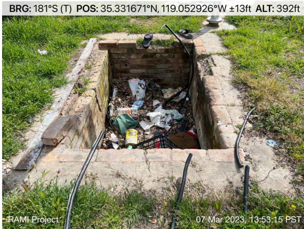
Photo 15. In-ground pit filled with garbage located on the southeast quarter of property in APN 441-382-04
