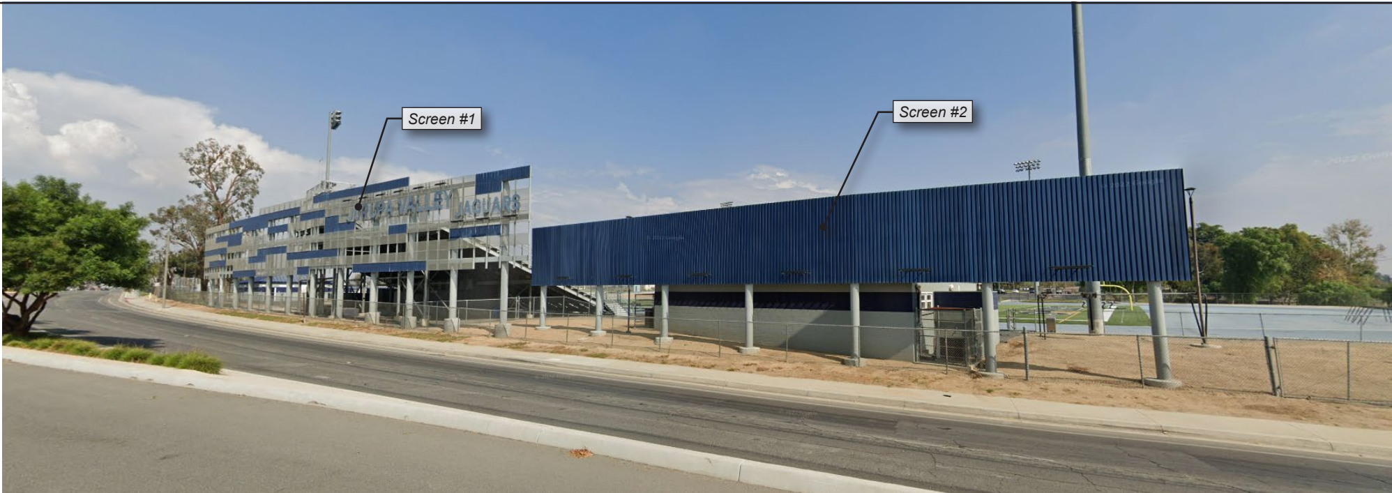
View of metal screen examples looking northeast from Etiwanda Avenue.
