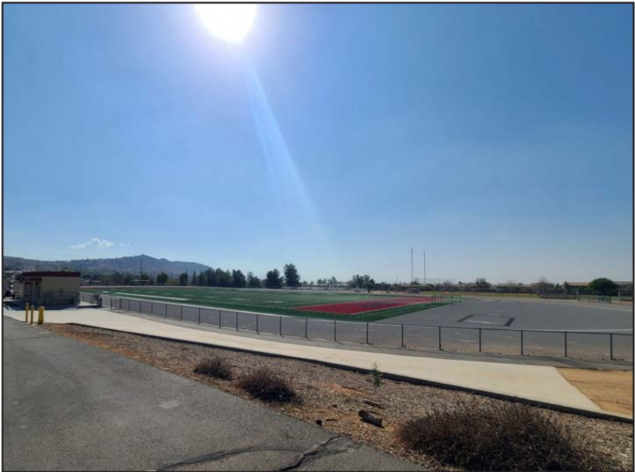
③ View 3: From the northeastern side of the track and field, looking southeast at the track and field on the project site.
