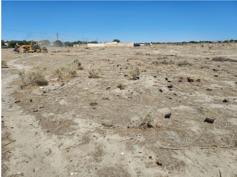
Figure 5 Project Area, Site R-6, Cultural Material with blade cut on the left and backhoe in the background
