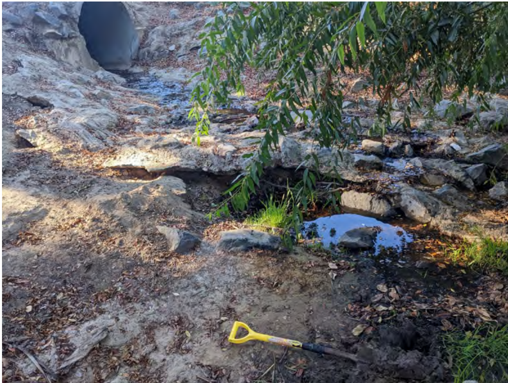
Photo 3: Wetland within the channel with grouted riprap, looking northwest.
