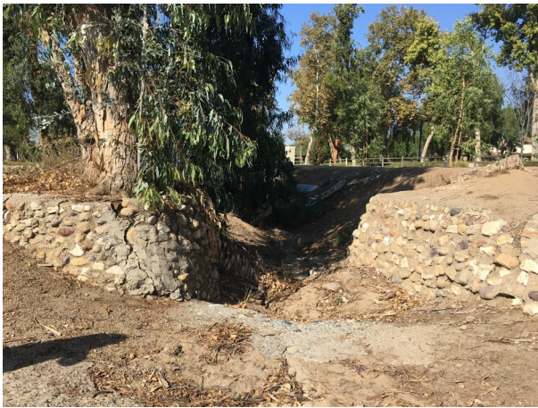
Creek crossing retaining walls, west perspective 10/28/2022; IMG_6118
