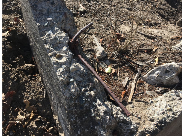
Check dam # 1, metal rebar, southwest perspective 10/28/2022; IMG_6107
