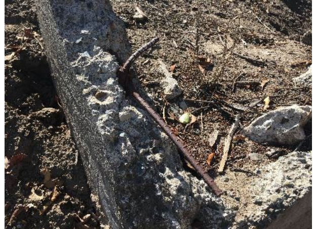
Plate 21. Check dam # 1, metal rebar (southwest perspective)
