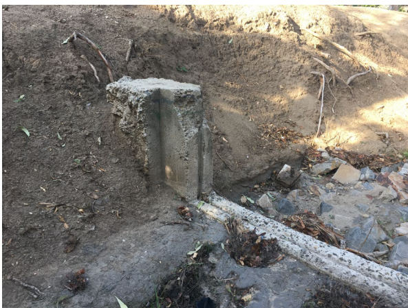
Check dam # 4, northeast perspective 10/28/2022; IMG_6058
