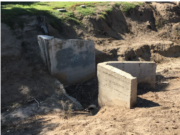
Check dam # 3, southwest perspective 10/28/2022; IMG_6201
