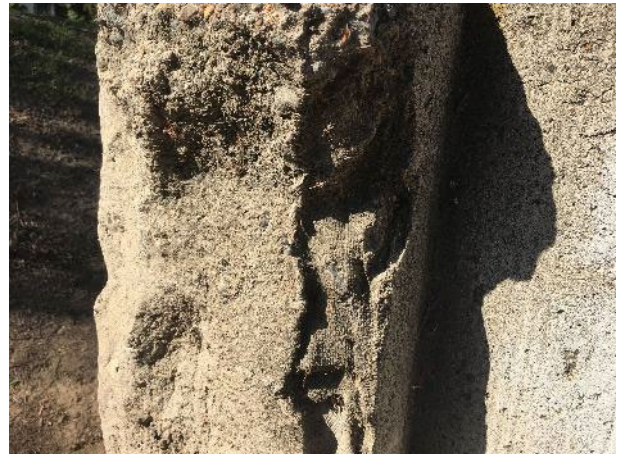
Plate 23. Check dam # 2, burlap imprint (northwest perspective)
