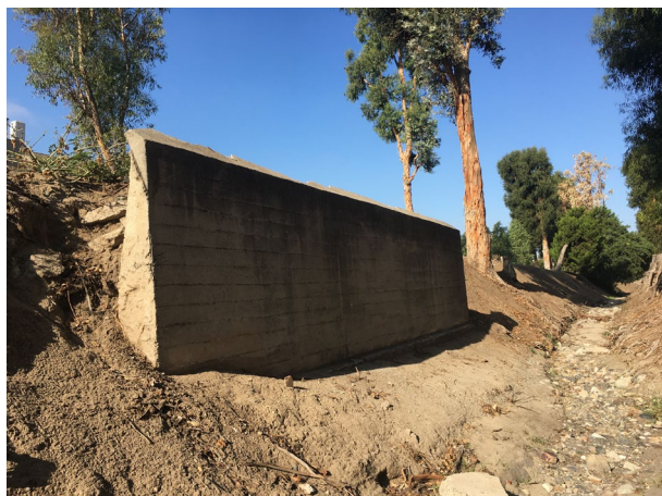
Concrete retaining wall, southwest perspective 10/28/2022; IMG_6063
