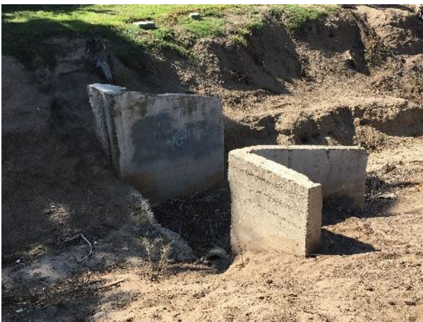
Plate 24. Check dam # 3 (southwest perspective)
