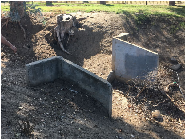
Check dam # 2, southeast perspective 10/28/2022; IMG_6095
