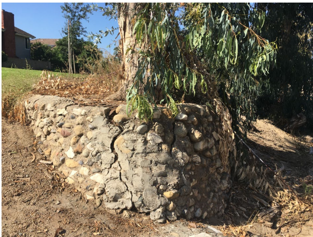
Creek crossing retaining walls, southwest perspective 10/28/2022; IMG_6117
