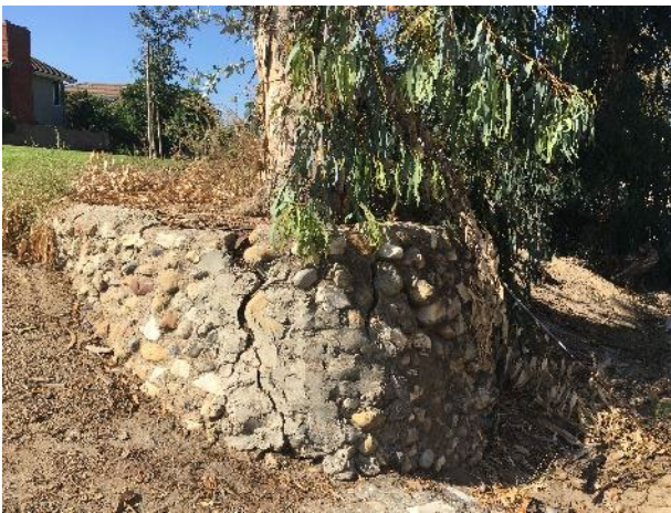
Plate 17. Creek crossing retaining walls (southwest perspective)
