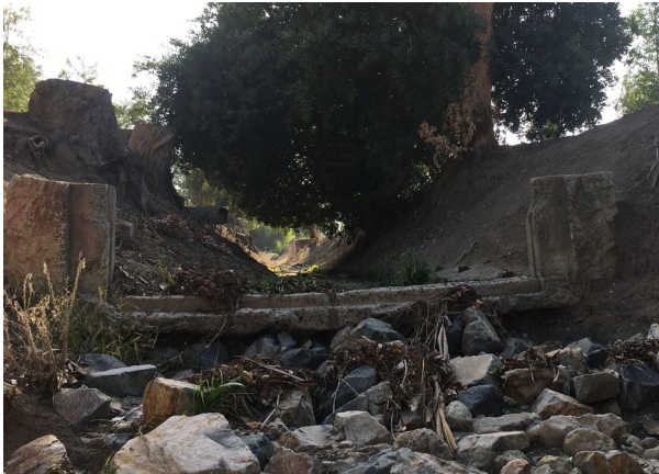
Check dam # 4, west perspective 10/28/2022; IMG_6054
