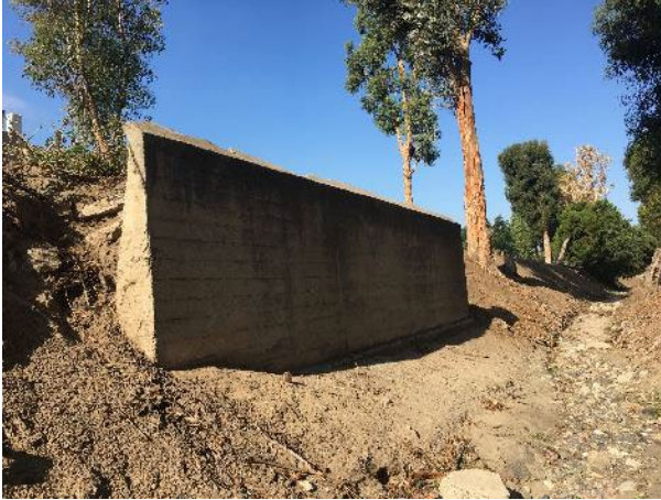
Plate 32. Concrete retaining wall (southwest perspective)
