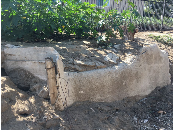
Gunit channel wall # 6, southwest perspective 10/28/2022; IMG_6169
