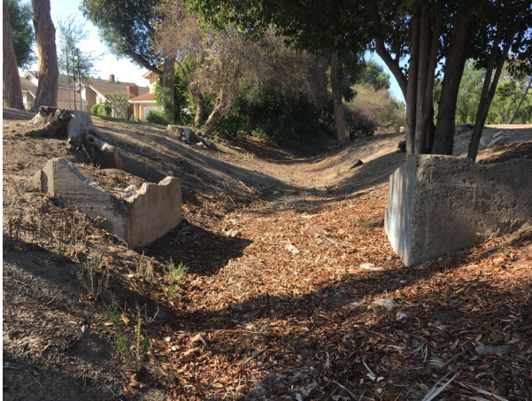
Check dam # 1, west perspective 10/28/2022; IMG_6108
