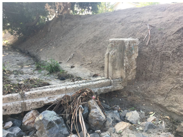
Check dam # 4, southwest perspective 10/28/2022; IMG_6056
