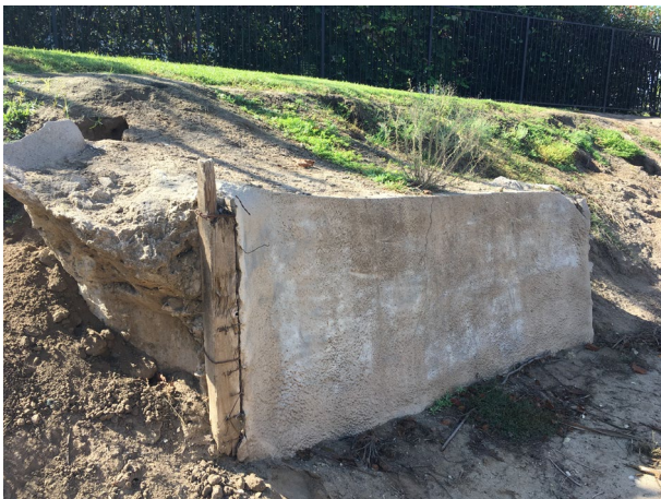
Gunit channel wall # 9, northeast perspective 10/28/2022; IMG_6147
