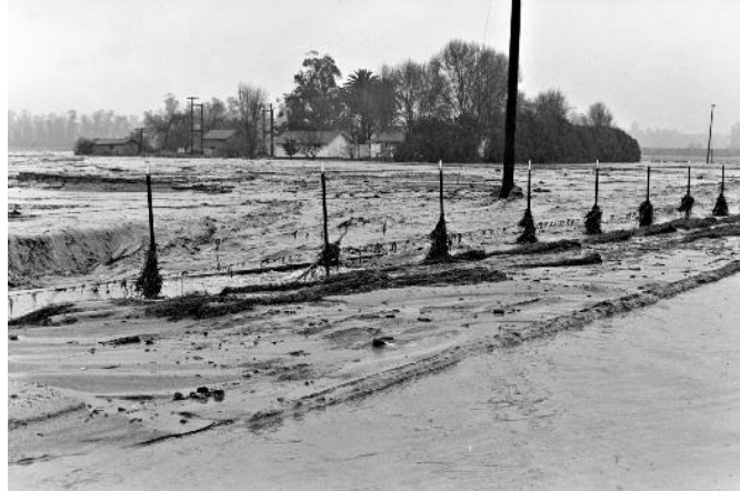
Plate 6. Storm damage along Rattlesnake Canyon Wash, 1969. Courtesy Orange County Archives
