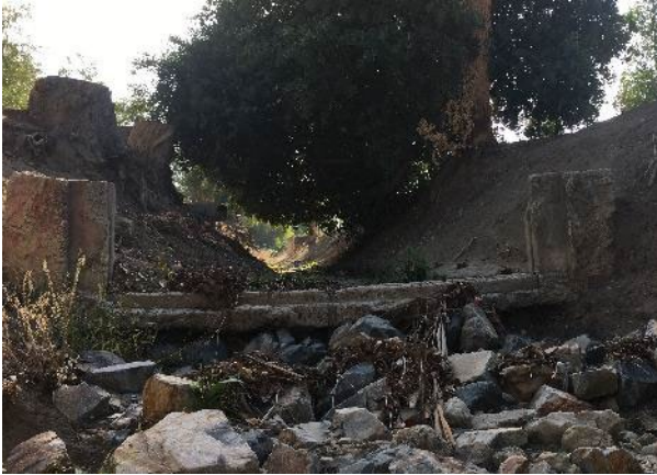
Plate 28. Check dam # 4 (west perspective)
