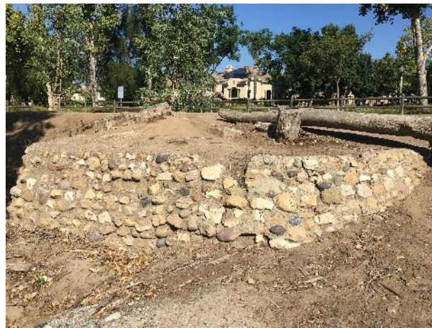
Plate 18. Creek crossing retaining walls (northwest perspective)
