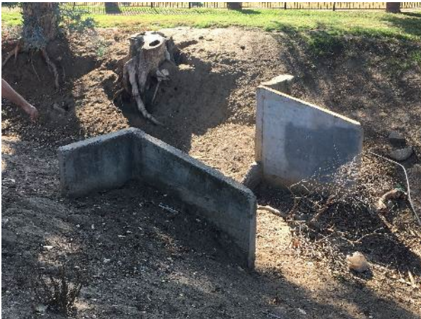
Plate 22. Check dam # 2 (southeast perspective)
