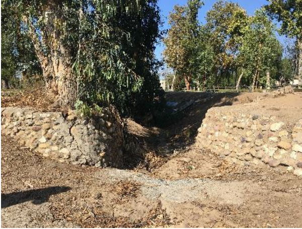
Plate 15. Creek crossing retaining walls (west perspective)
