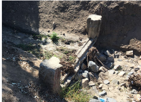
Check dam # 4, southwest perspective 10/28/2022; IMG_6203
