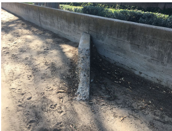
Concrete sidewalk wall, fragment, southeast perspective. 10/28/2022; IMG_6072
