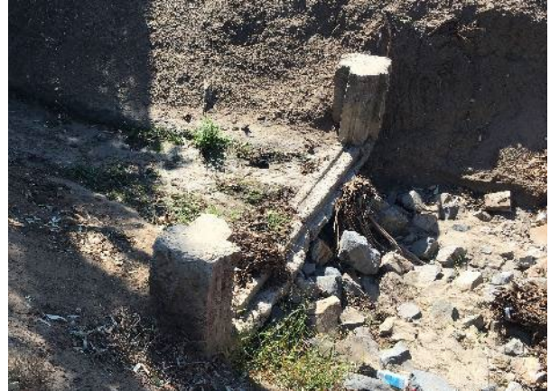
Plate 29. Check dam # 4 (southwest perspective)
