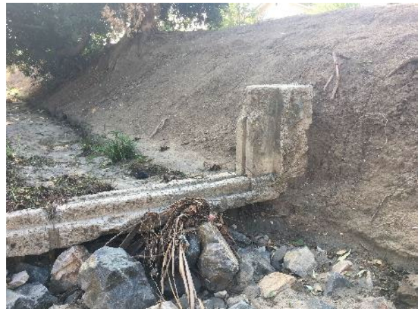
Plate 31. Check dam # 4 (southwest perspective)
