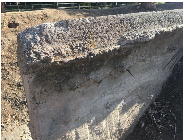
Concrete retaining wall, fragment, northeast perspective 10/28/2022; IMG_6064
