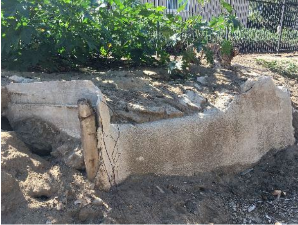
Plate 7. Guniting channel wall #6 (southwest perspective)
