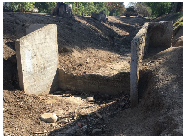
Check dam # 3, northeast perspective 10/28/2022; IMG_6091
