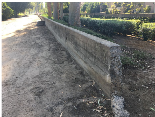
Concrete sidewalk wall, southeast perspective 10/28/2022; IMG_6073
