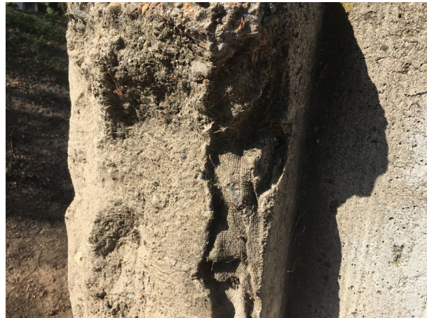
Check dam # 2, burlap imprint, northwest perspective 10/28/2022; IMG_6098
