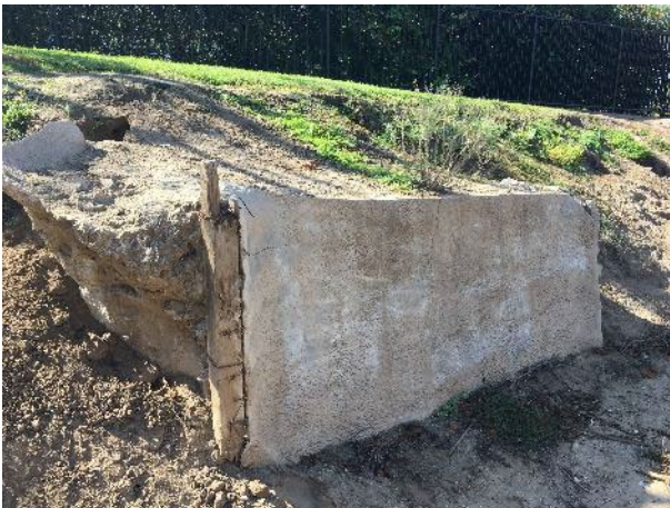
Plate 9. Guniting channel wall #9 (northeast perspective)
