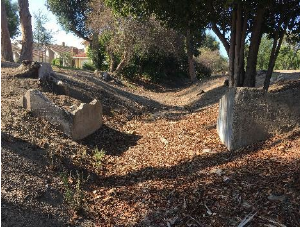
Plate 20. Check dam # 1 (west perspective)
