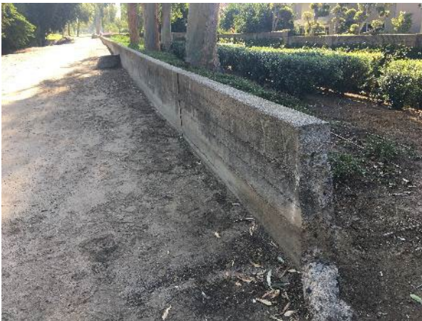
Plate 34. Concrete sidewalk wall (southeast perspective)
