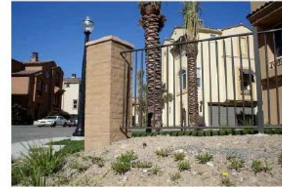
— Tubular Steel Fence with Slump block pilasters per plan
