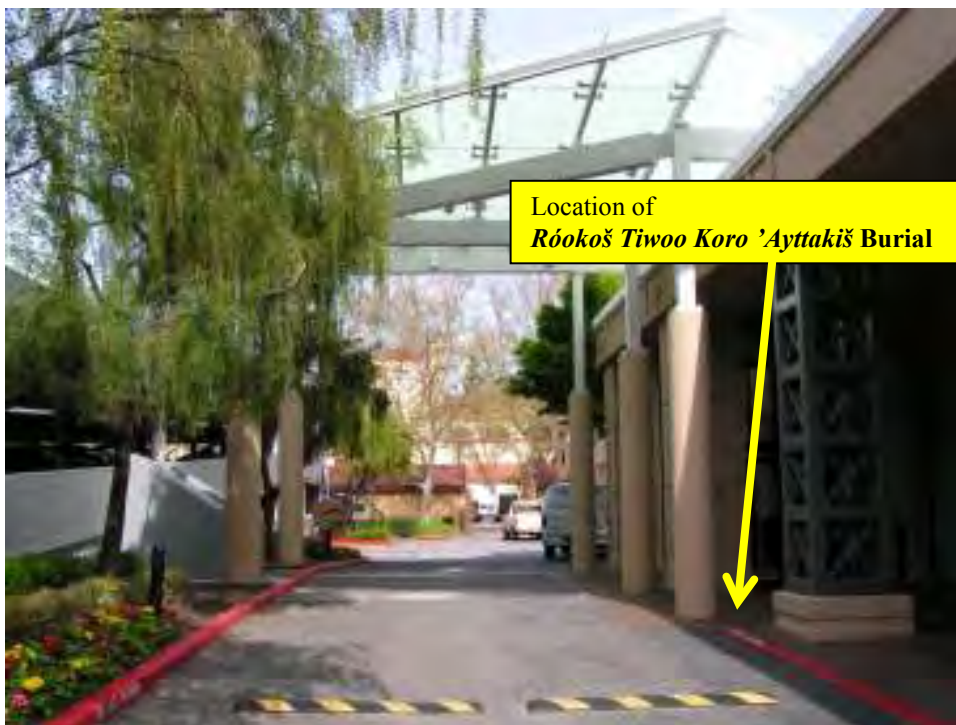
Figure 3-19: View Looking East of the Finished Support Columns and Canopy
