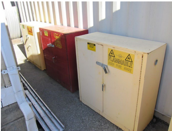
Photograph 5. Flammable material storage cabinets at corporation yard (Parcel 5).
