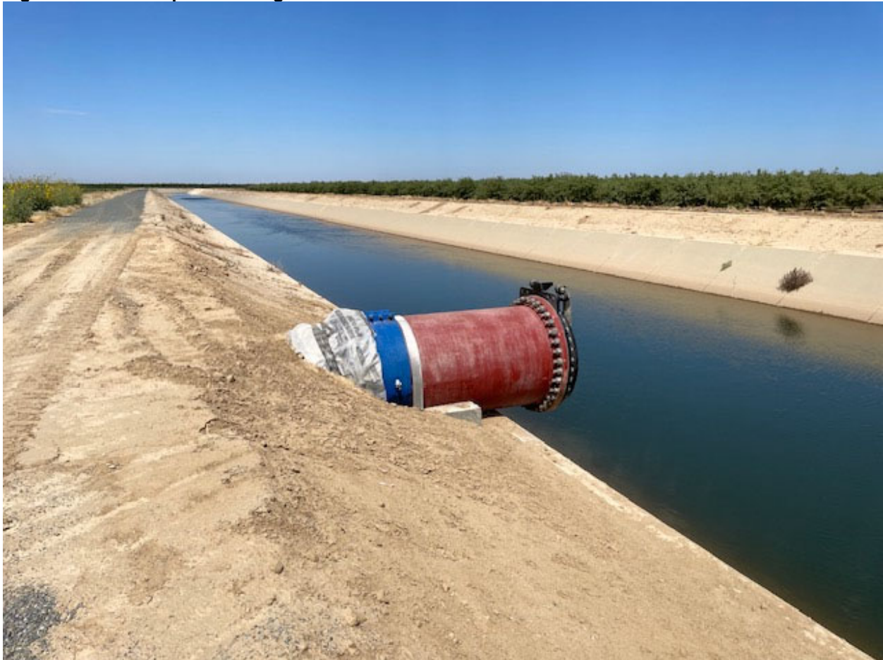
Figure 2-4. Example Discharge Outfall.
