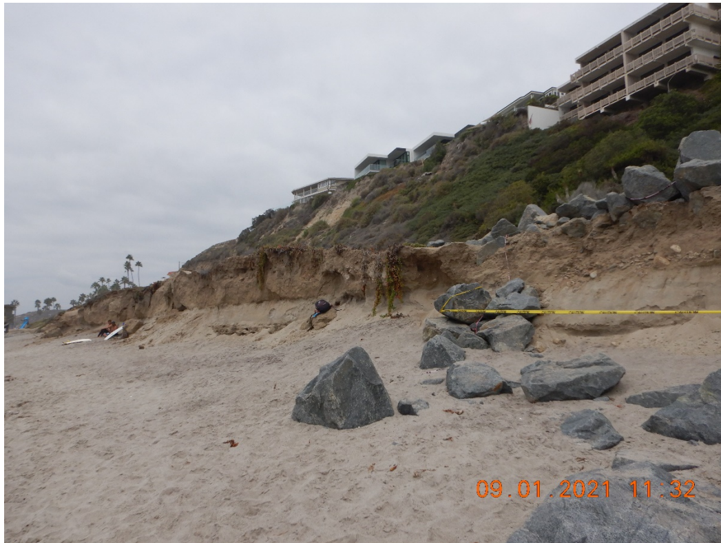
Damage to Earthen Berm
