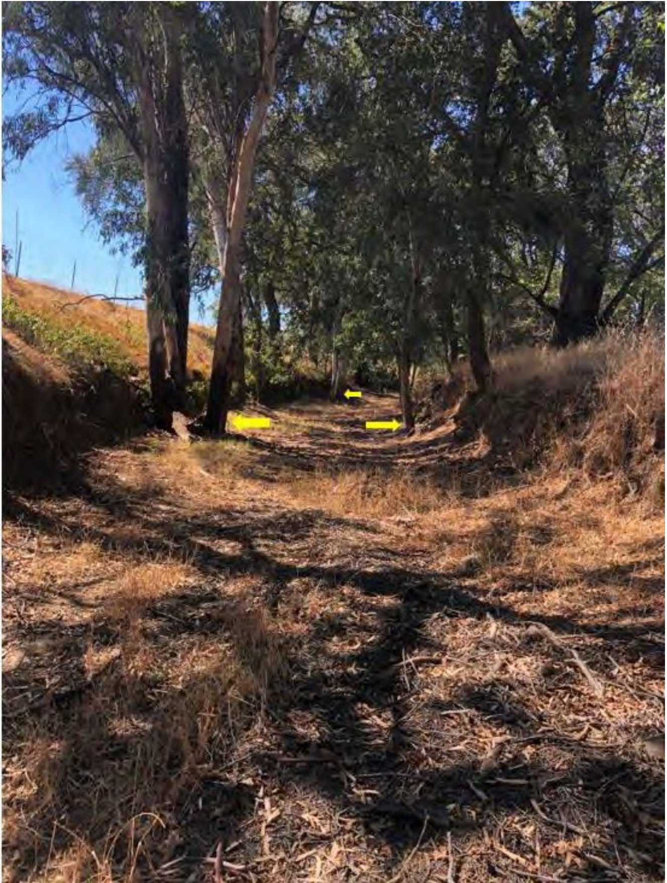
Figure 9. Typical view of Grasshopper Slough channel, non-native trees to be removed in the low flow channel (yellow arrows) and levee erosion repair area on the left.
