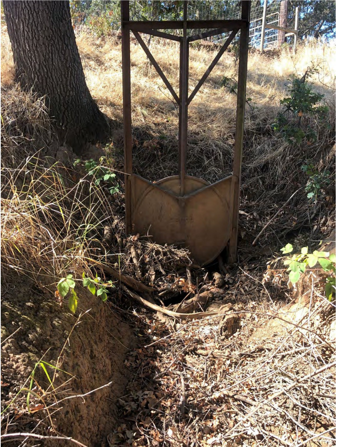
Figure 10. View of a culvert pipe to be abandoned in order to preserve surrounding mature oak trees.
