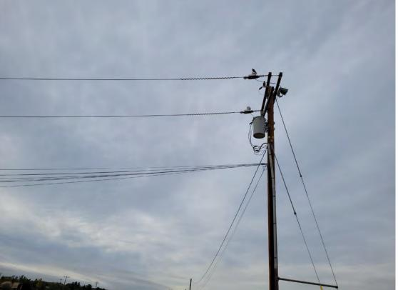
Photograph Number 4: Pole-mounted transformer
