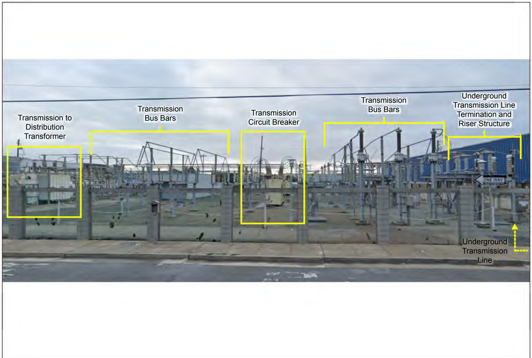
Figure 2-3 Examples of Aboveground Infrastructure at an Electrical Substation
