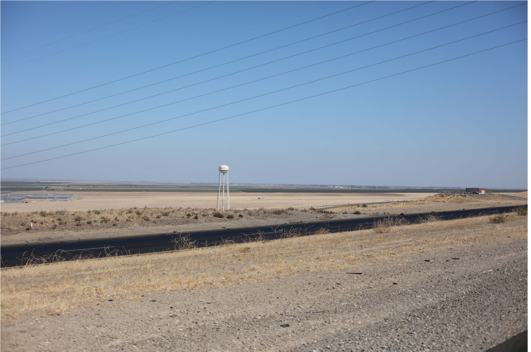
a) View to the east-southeast from KOP 3. The Mercy Springs Substation, just west of the Vega Solar Project and visible along the left edge of this view, is 0.8 mile east of this segment of southbound I-5. The Dos Amigos Pumping Plant facilities along the right edge of the view are about 0.33 mile to the east.
