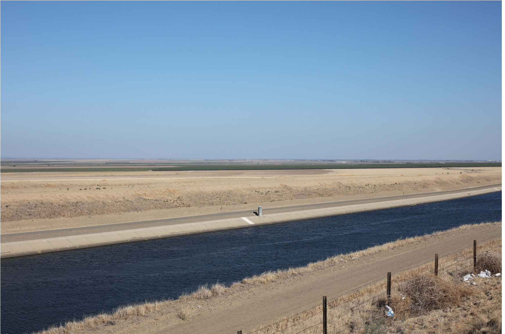
a) View to the east-southeast from KOP 2. The California Aqueduct in the immediate foreground is located approximately 0.05 mile east of the Dos Amigos Pump Station Vista Point. The orchard in the center of the view is as close as 1.5 miles away to the east-southeast.
