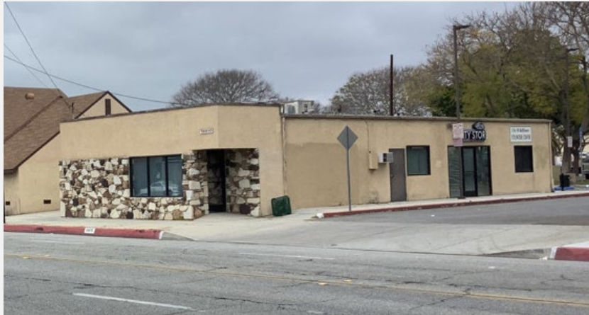
Exhibit 2. West and primary (south) elevations of the Municipal Storage Building, view looking northeast.
