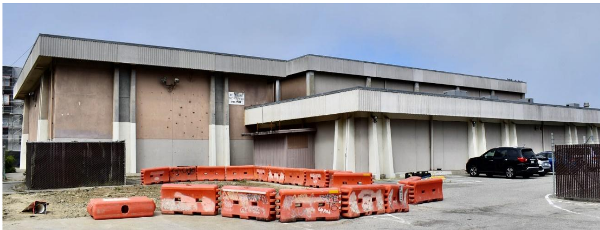
Figure 5 Gymnasium, South Side, View North
