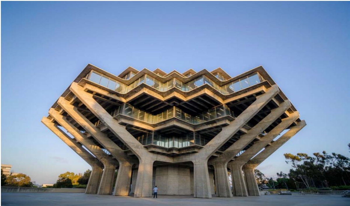
Figure 20 Geisel Library, University of California at San Diego. Photo: University Communications, UC San Diego
