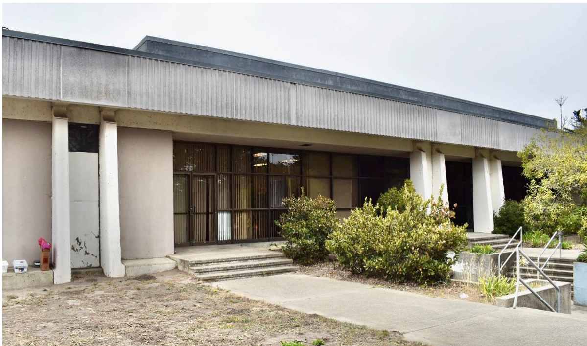
Figure 8 Cafeteria Wing, Looking Southwest
