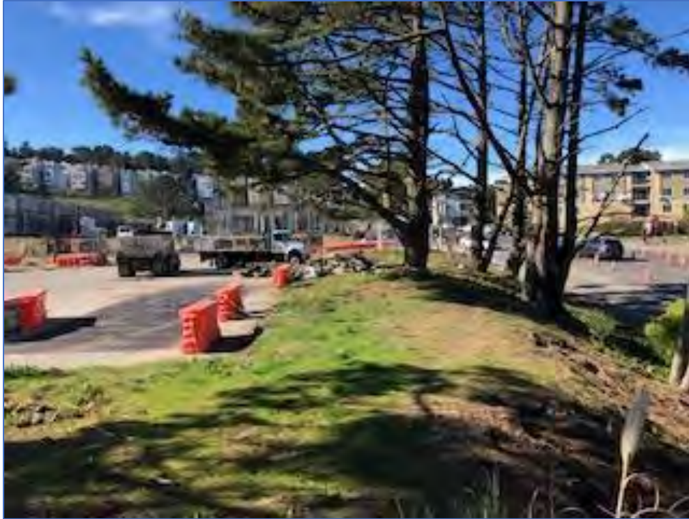
View 3. View to west along Serramonte Blvd frontage of dense mature with new construction in northwestern portion of the site.
