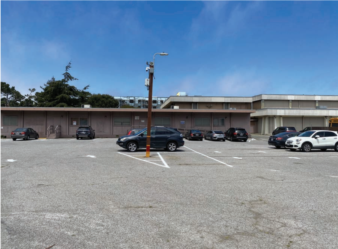
Photo 3: View of administration building looking north.
