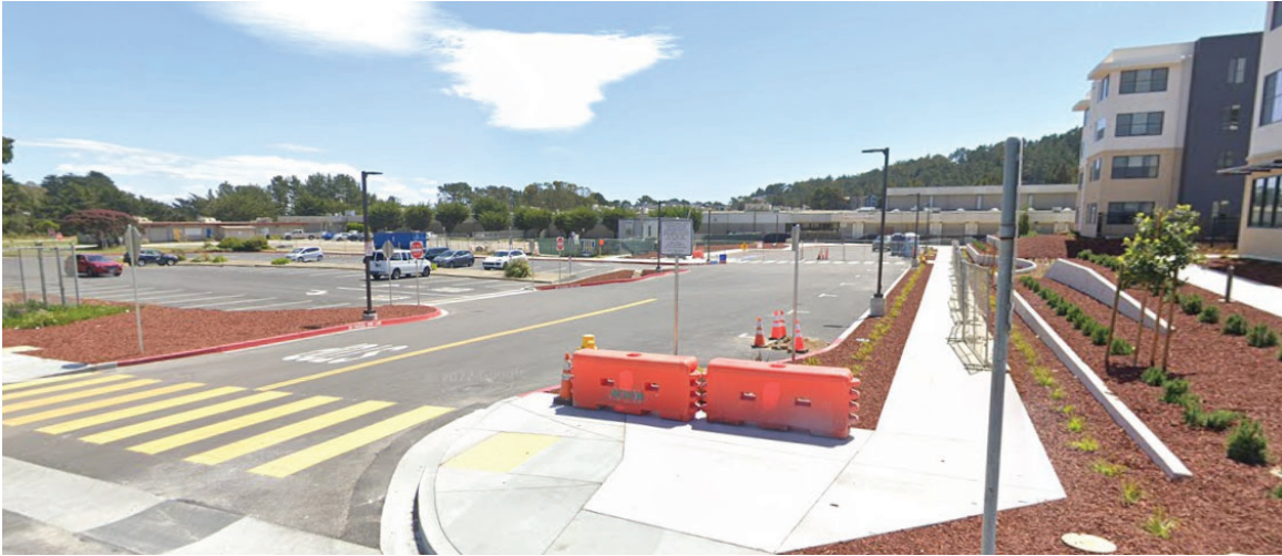
Photo 1: View from Serramonte Boulevard looking south.
