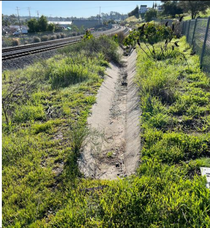
Photograph 9: (33.196593 N, -117.240733 W) Southeast-facing view of the one-foot-wide Channel 3 along the eastern edge of the survey area. This photo shows where Sampling Point NW-3-1 was taken to determine the presence of OHWM indicators. The northern extent of the concrete-lined channel is also visible in the lower-half of the photo.
