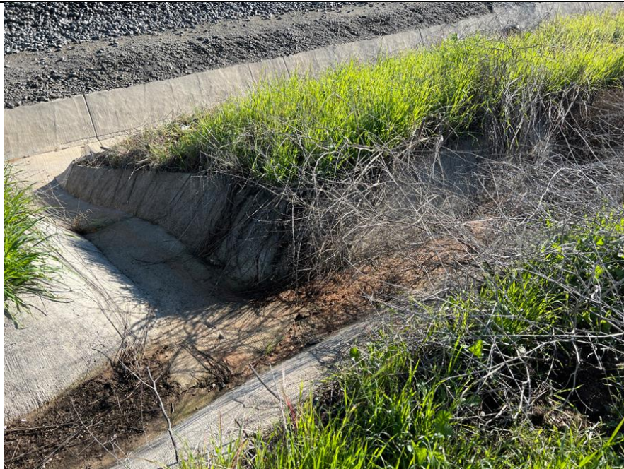
Photograph 10: (33.196412 N, -117.240628 W) East-facing view of Channel 3 along the eastern edge of the survey area. This photo shows where Channel 3 connects to another larger concrete-lined channel that runs parallel east of the survey area through the SPRINTER transportation right-of-way.
