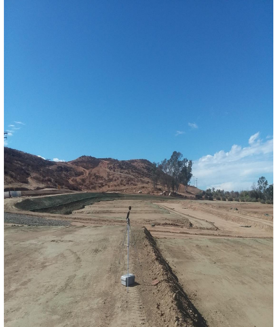
NM1 looking West parallel to Garbani Road
