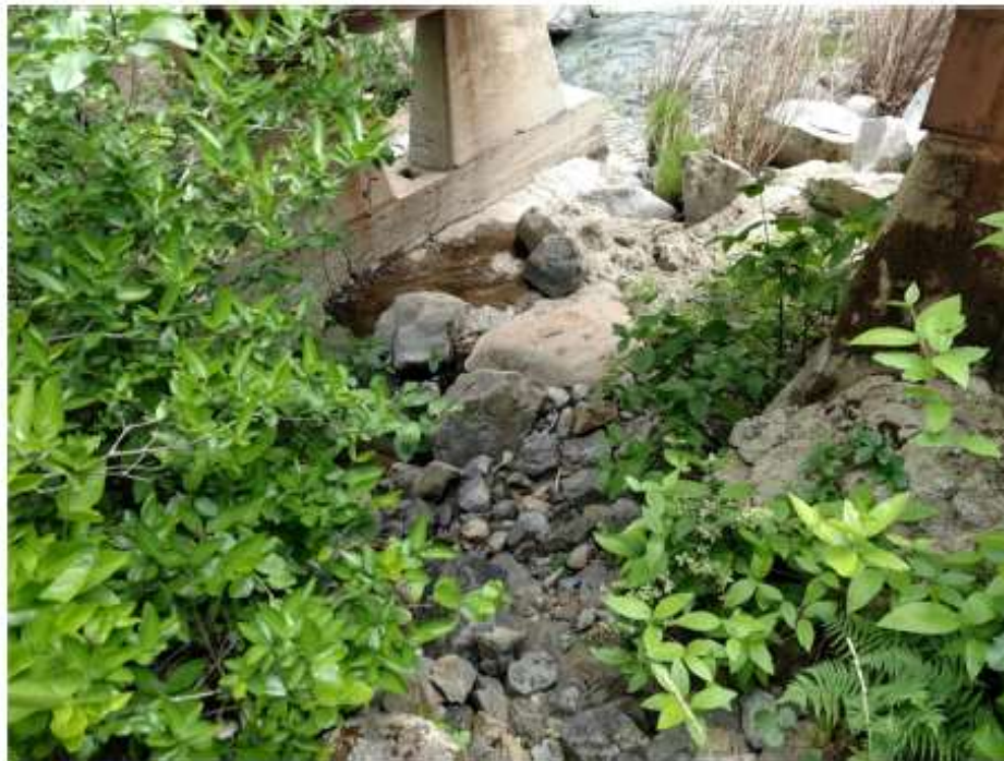
View of Moss Creek channel underneath Moss Canyon Bridge, below the OHWM (photo facing northeast). Note the concrete in the active channel underneath the bridge.
