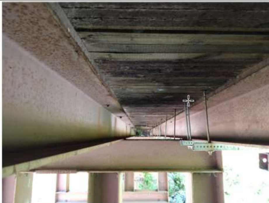
View underneath Moss Canyon Bridge. The bridge may provide nesting opportunities for migratory birds, but gaps in timber decking are too wide to provide refuge for roosting bats. (photo facing west)
