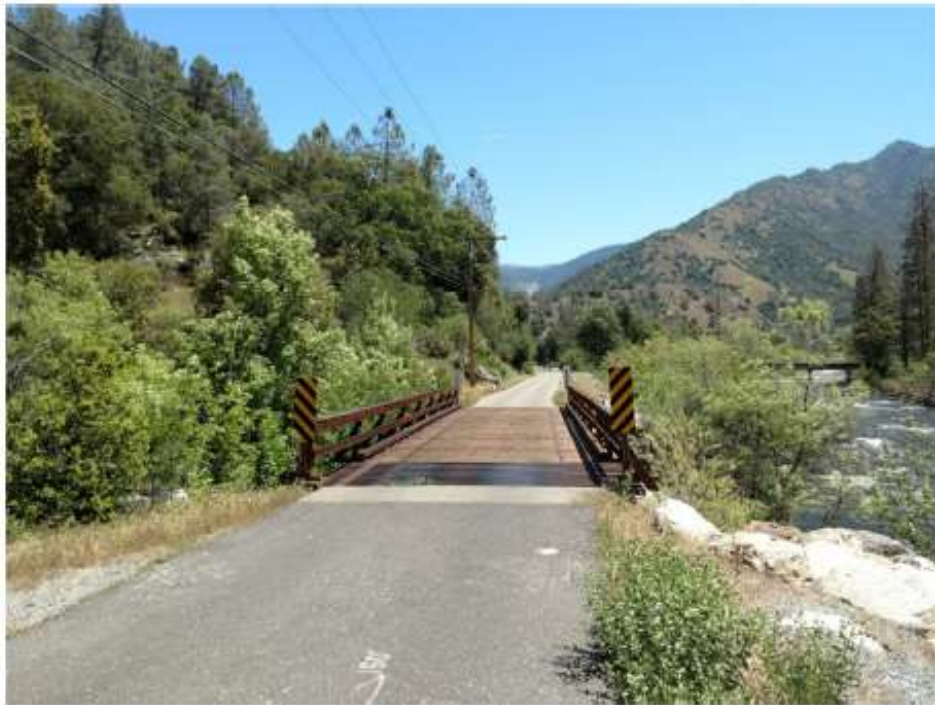
Moss Canyon Bridge along Incline Road marks the confluence where Moss Creek (located north [left] of the bridge) connects to the Merced River (located south [right] of the bridge) (photo facing east).
