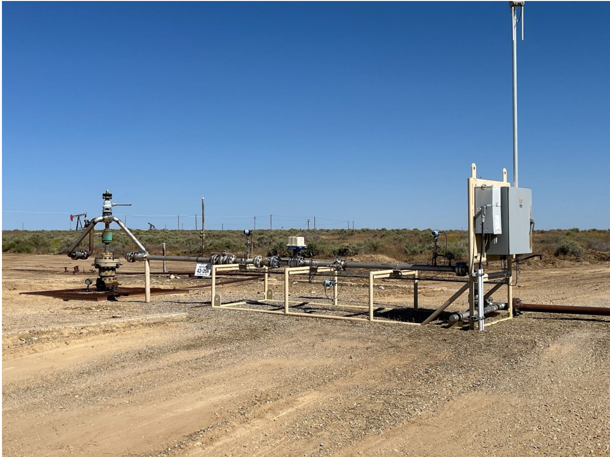
Figure 4.1-17: Existing Water Injection Well (CLASS VI UIC CO 2 Injection Well would look similar)
