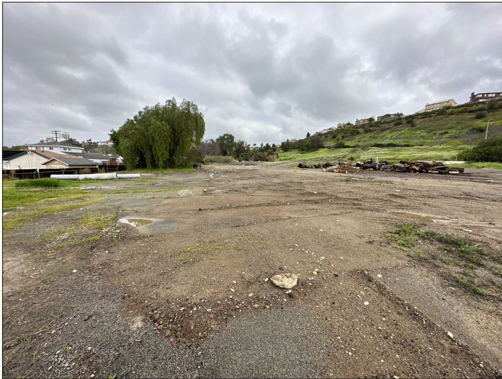
Photo 1: View from south end of project area looking north/northwest showing unvegetated central site. Photo taken on March 16, 2023.
