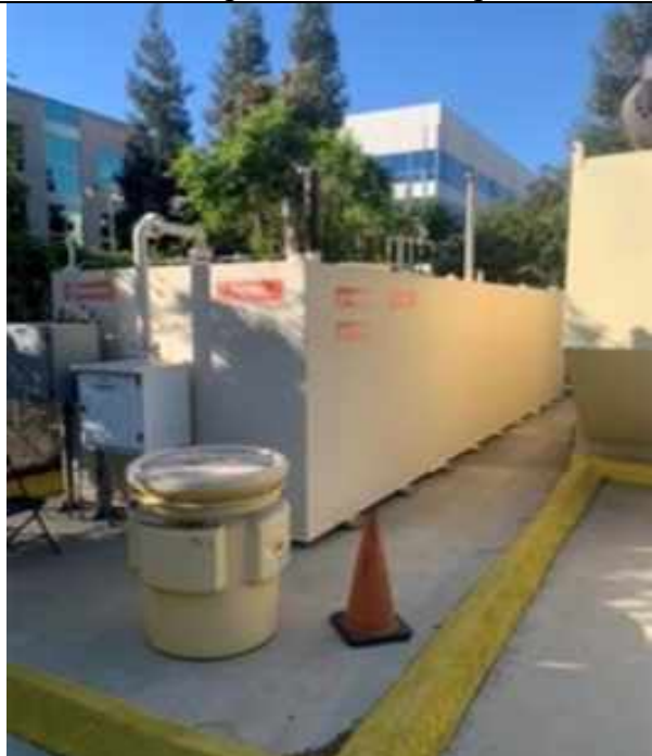
10,000 gallon AST on the northern parcel in a secondary containment dyke.
