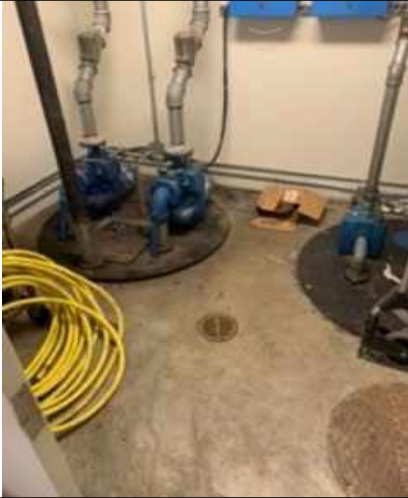
Sump pump units in the basement of the Broadcast building on the northern parcel.
