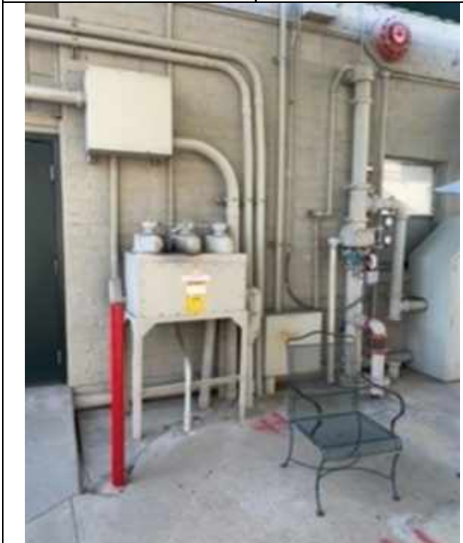
One of four electrical switches that are labeled as containing PCBs.
