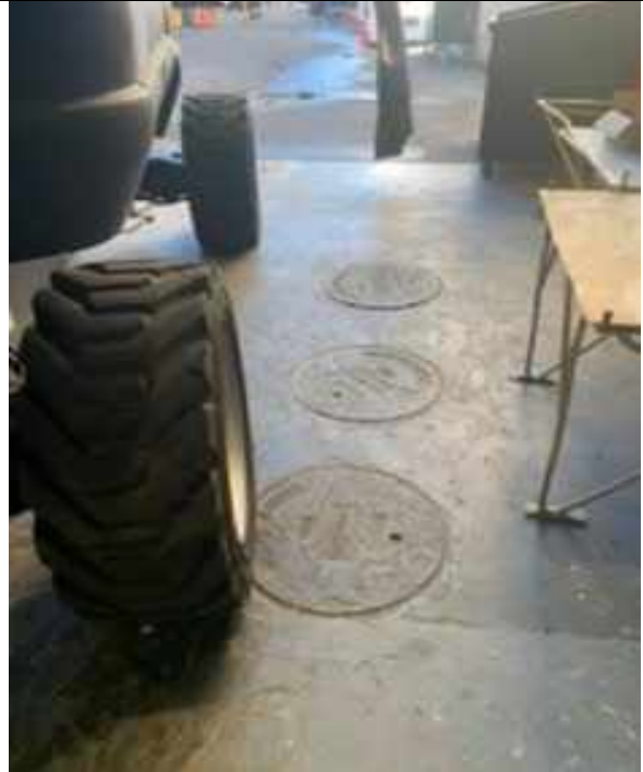
Access manholes to a clarifying tank unit in the Paint Shop on the southern parcel.
