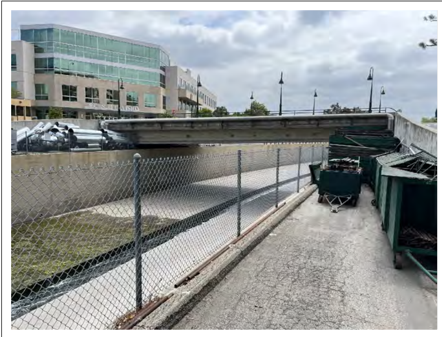
Photo Location 3, facing northeast. June 2, 2023. View of western side of bridge to be expanded over Los Angeles River. Note the bridge footings are located above the concrete side levee of the river.
