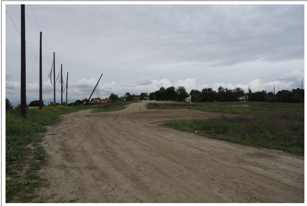
Photo 3 - Taken from the west part of the Project site looking northeast.
