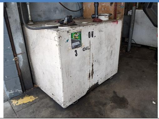
**PHOTO 15:** View of the 250-gallon motor oil AST at Service Bay D.
