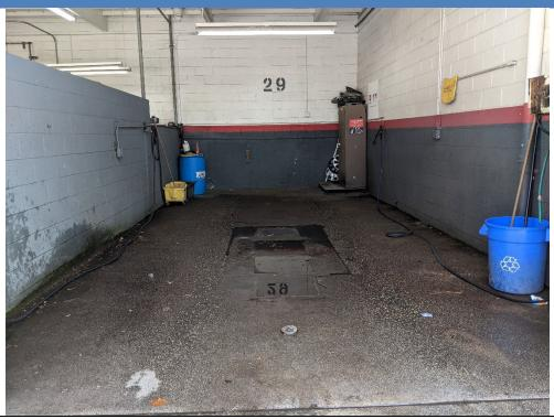
**PHOTO 13:** View of the car wash area and clarifier at Service Bay D, looking south.
