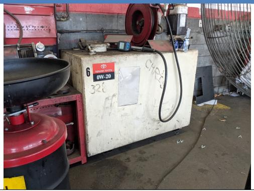
PHOTO 11: View of the 250-gallon motor oil AST at Service Bay C.
