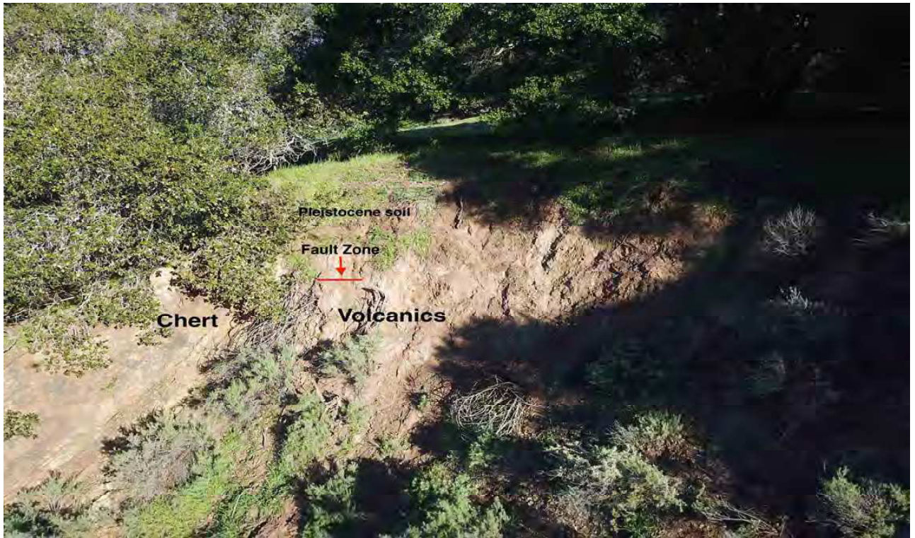
Looking north at the northern cut for the parking lot. Chert bedrock is on the left and Volcanic rocks (tuff) is on the right. The fault is in the center.
