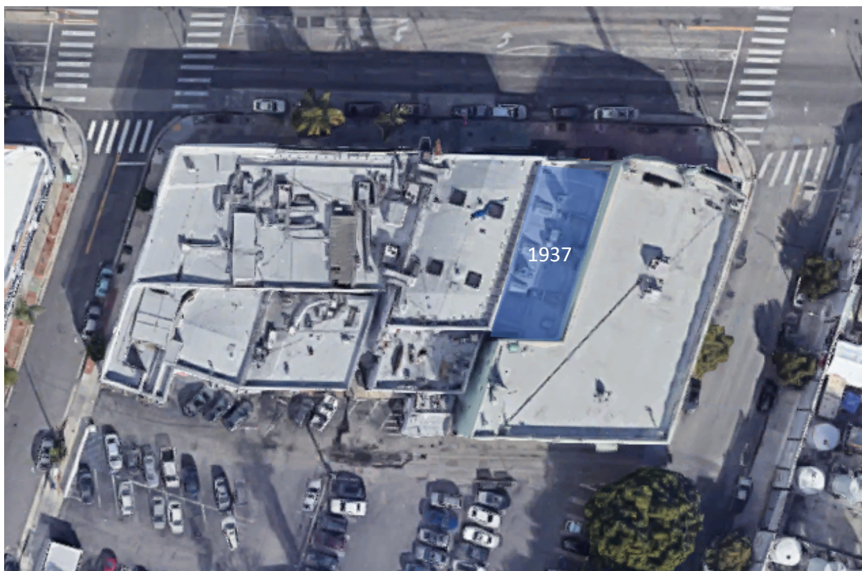
Figure 15: Project Site, 5354-56 Wilshire Boulevard shaded in blue.
