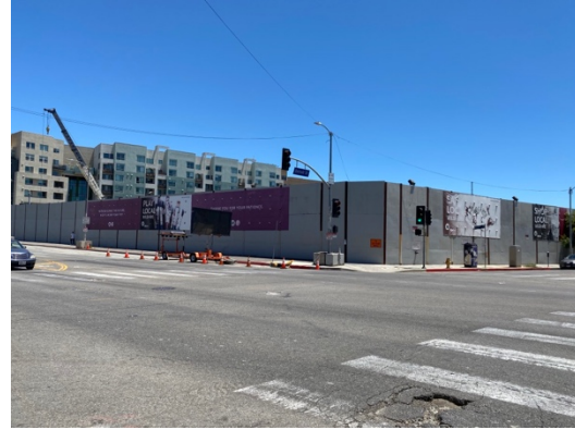
Figure 20: 5320-40 Wilshire Boulevard, July 2022, TGHP.
