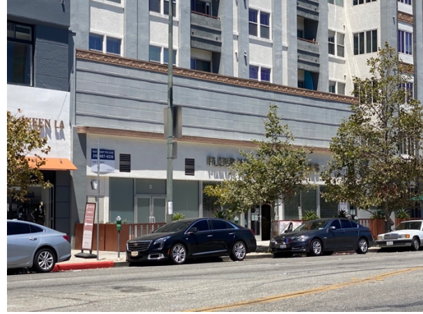
Figure 22: 5355-59 Wilshire Boulevard, July 2022, TGHP.
