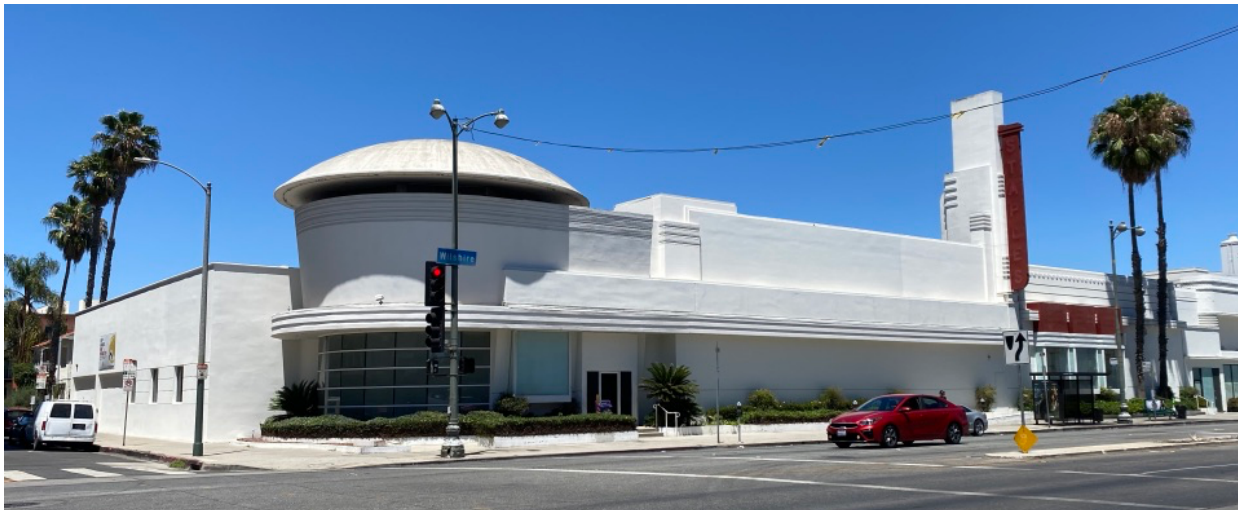
Figure 25: 5413-15 Wilshire Boulevard, July 2022, TGHP.
