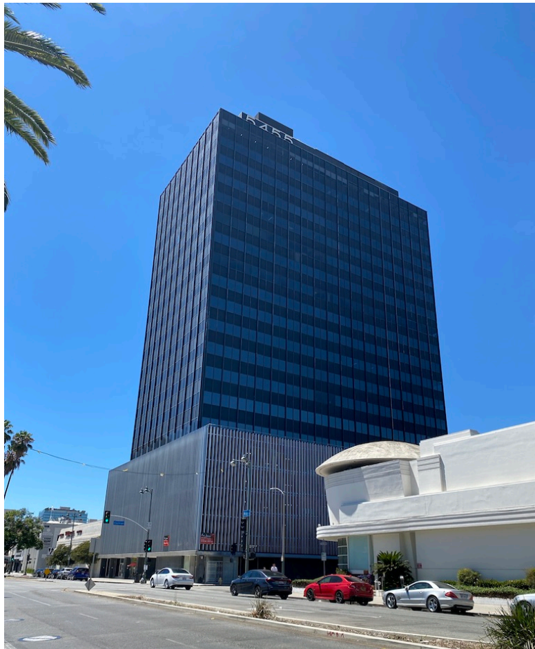
Figure 26: 5455 Wilshire Boulevard, July 2022, TGHP.
