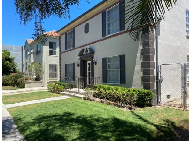
Figure 46: View looking northeast on Detroit Street from mid-block, July 2022, TGHP.
