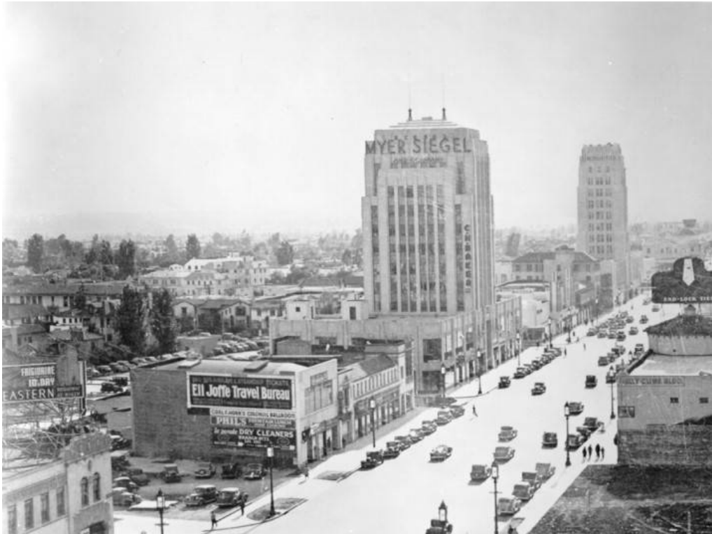
Figure 11: View looking southwest from Wilshire Boulevard and La Brea Avenue, 1932, Los Angeles Public Library Photograph Collection.
