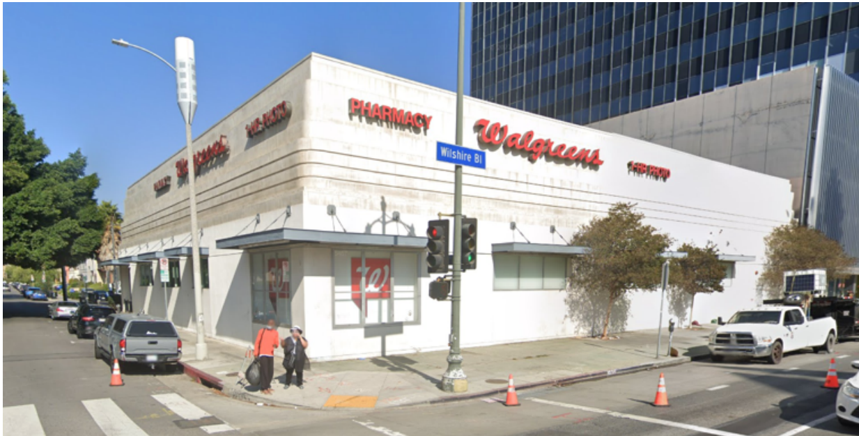
Figure 29: 5465-69 Wilshire Boulevard, July 2022, TGHP.
